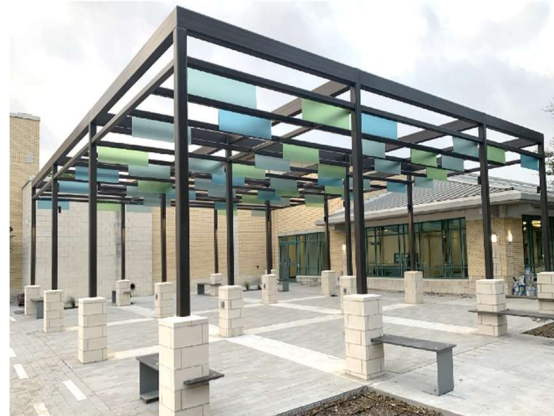
Panels Installed on Trellis at Alumni Hall
