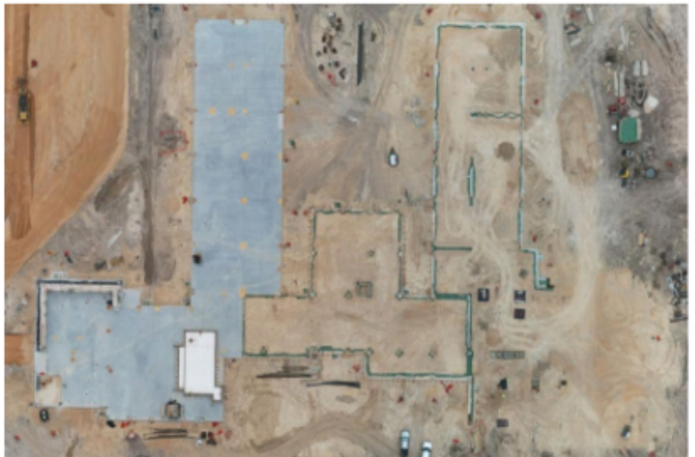
Aerial View of Building Pad
