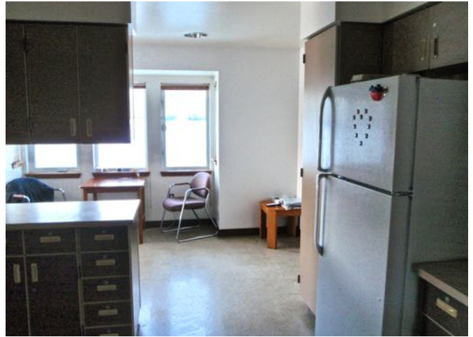
Back side of kitchen divider wall
