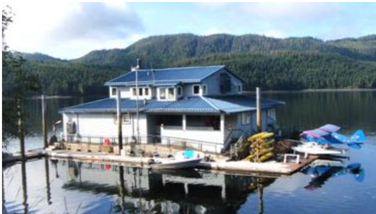
Overall view of North and East sides of subject
