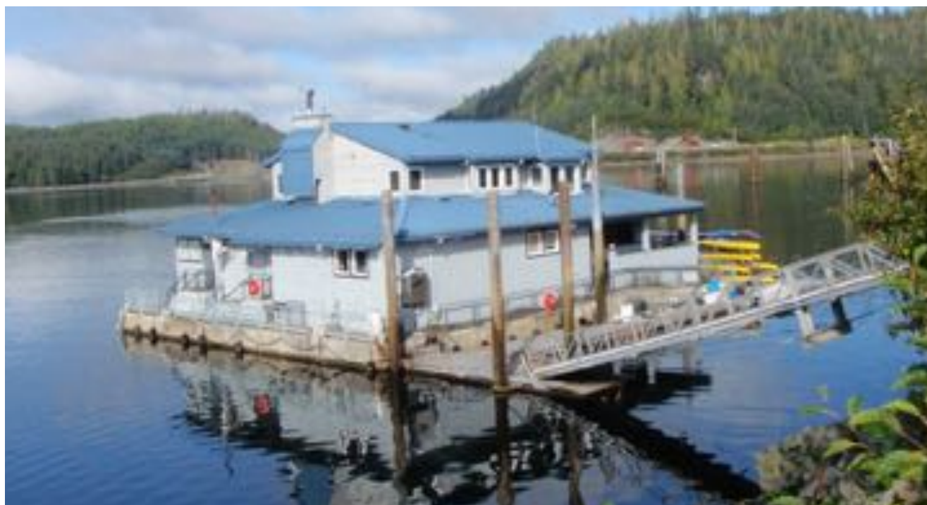
Overall view of Southeast corner of subject and gangway
