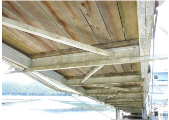
Access ramp (gangway) top side viewed from float and underside viewed from shore
