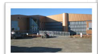
ALASKA TECHNICAL CENTER
