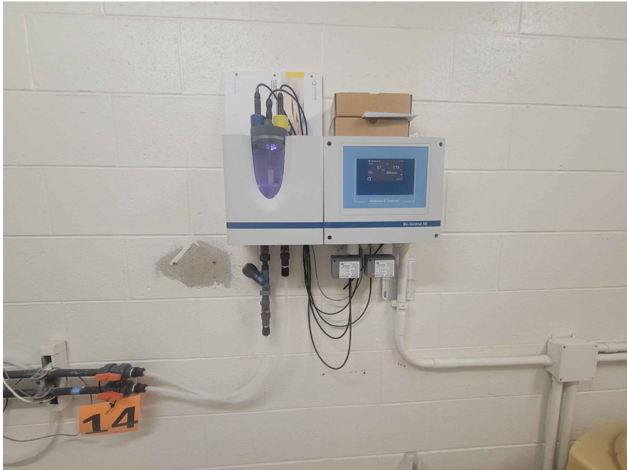
2 AQ0.3 EXISTING CHEMICAL CONTROLLER NTS
