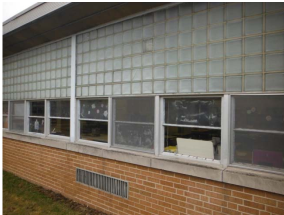
Photo #69: Original (200 & 300 wings) sections of building have original single-pane windows
