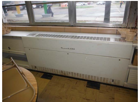
Photo #46: Horizontal unit ventilator in original building classroom
