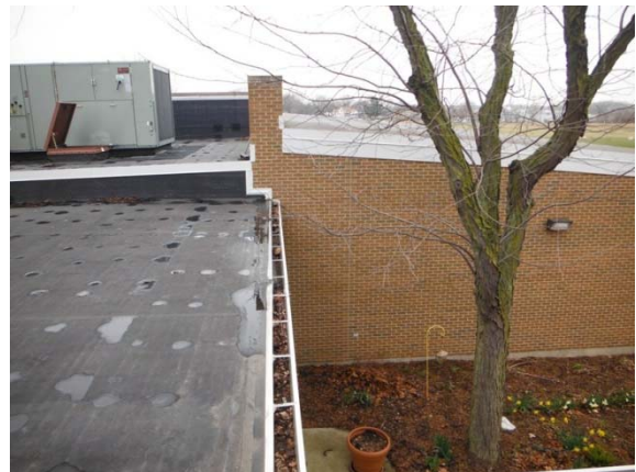
Photo #66: Clogged gutter on north side of building
