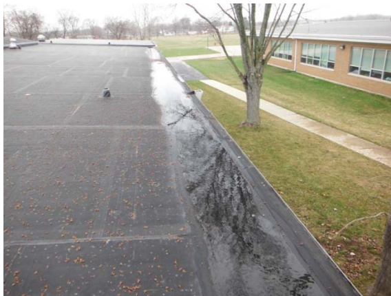
Photo #65: Ponding along north side of 200 wing roof
