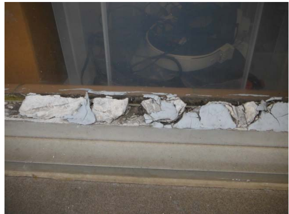
Photo #70: Close up of condition of single-pane windows
