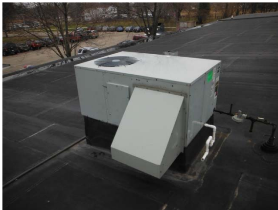
Photo #53: Gas-fired RTU for main office area
