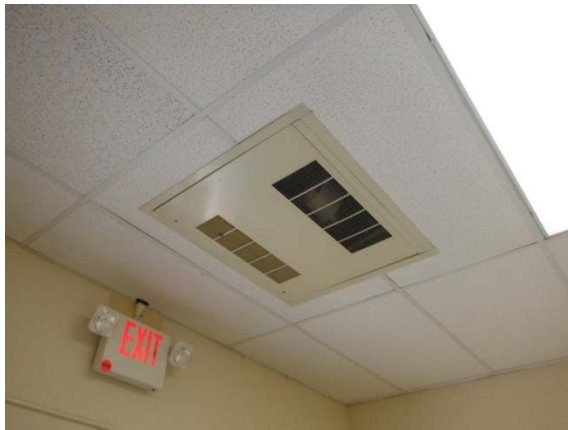
Photo #51: Common area fan coil unit above entrance door
