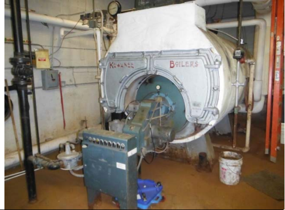
Photo #38: HVAC boiler in original section of building
