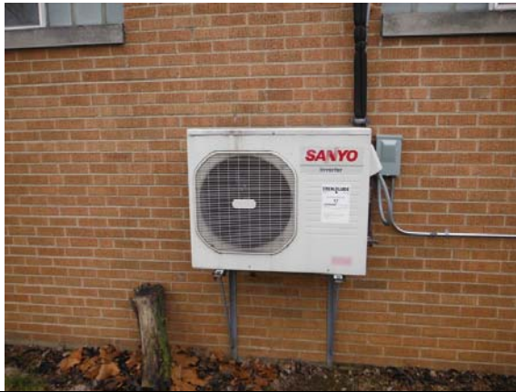
Photo #49: Ductless split system condenser for Parent liaison office
