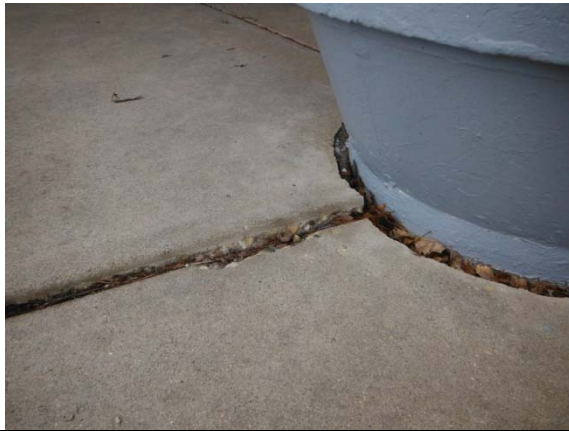
Photo #73: Concrete sidewalk settlement and open gaps at front walk
