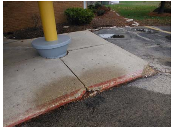
Photo #72: Spalling concrete sidewalk at front walk
