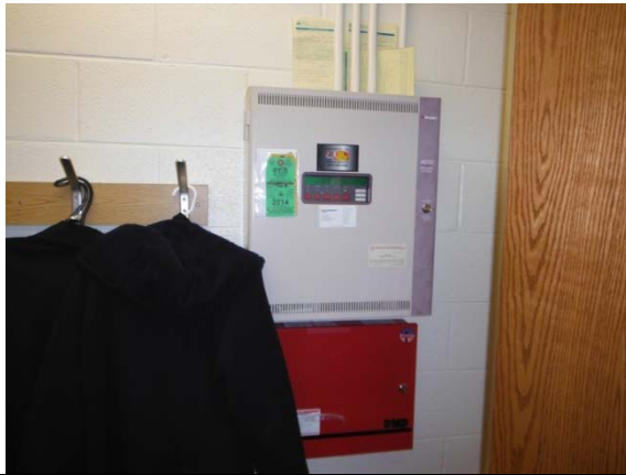
Photo #61: Central fire alarm panel
