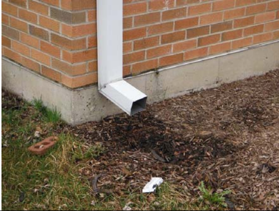
Photo #79: Missing splashblock at base of downspout at north side of building
