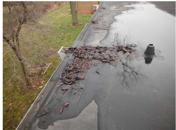
Photo #64: Clogged scupper and ponding on east side of 300 wing roof
