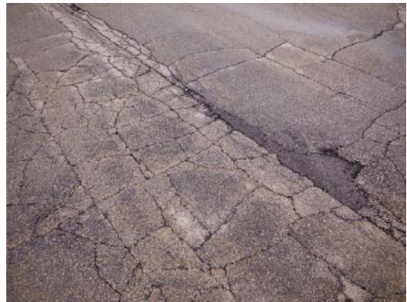
Photo #76: Asphalt deterioration at entry drive
