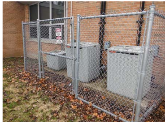
Photo #48: Condensers for Computer lab, Learning center and office area
