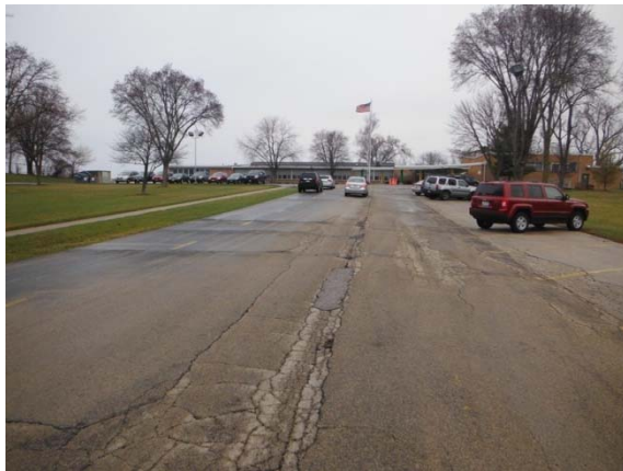
Photo #75: Condition of asphalt pavement at entry drive
