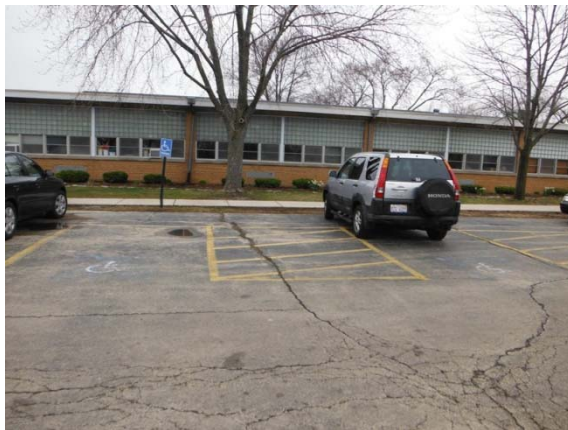
Photo #11: Accessible parking stalls –no van stalls and one vertical sign missing
