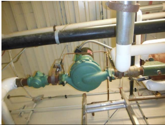
Photo #43: HVAC circulation pump
