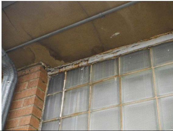
Photo #67: Rusting window framing at original section of building
