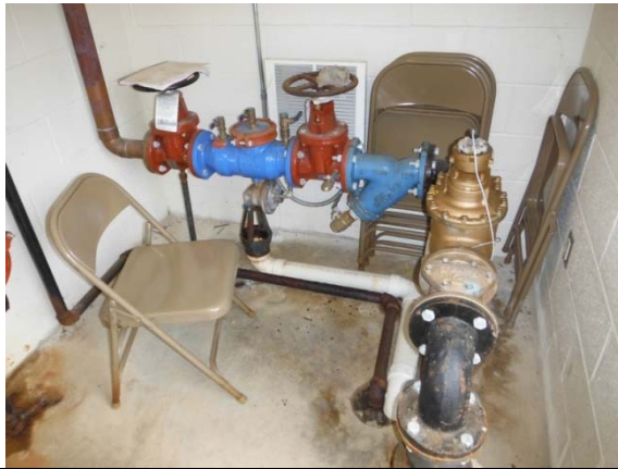
Photo #55: Domestic water backflow preventer and water meter
