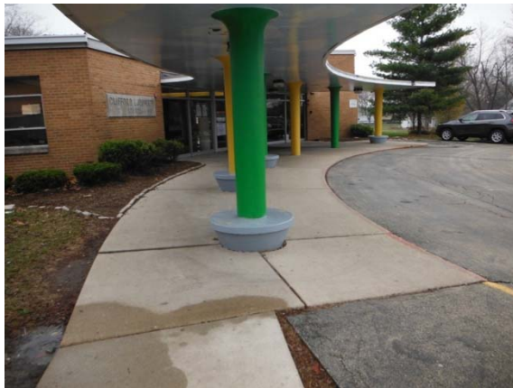
Photo #71: Minor settlement of concrete sidewalk at front walk
