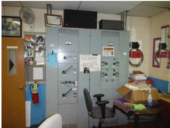
Photo #59: Main electrical switchboard
