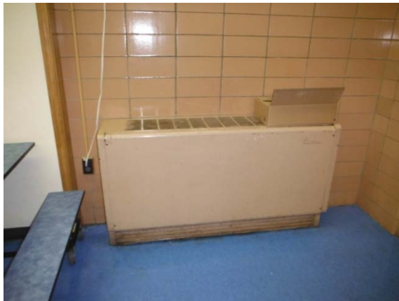
Photo #45: Horizontal unit ventilator in cafeteria
