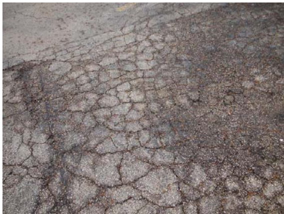
Photo #77: Asphalt deterioration at top of entry drive
