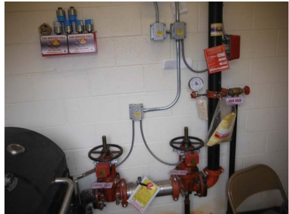
Photo #60: Sprinkler riser
