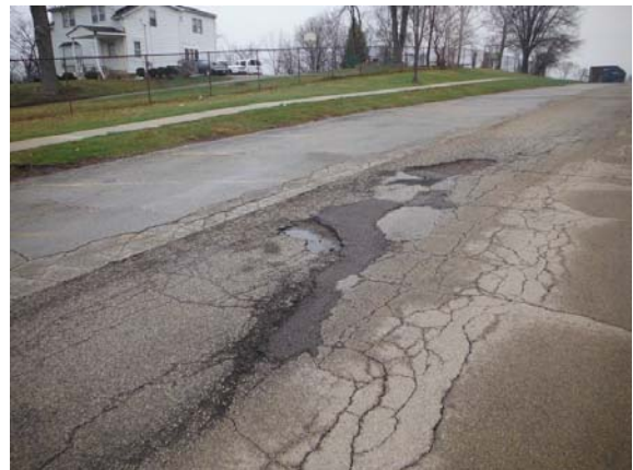
Photo #78: Asphalt deterioration at exit drive
