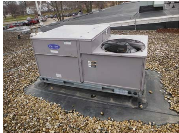
Photo #52: Electric RTU for main office area
