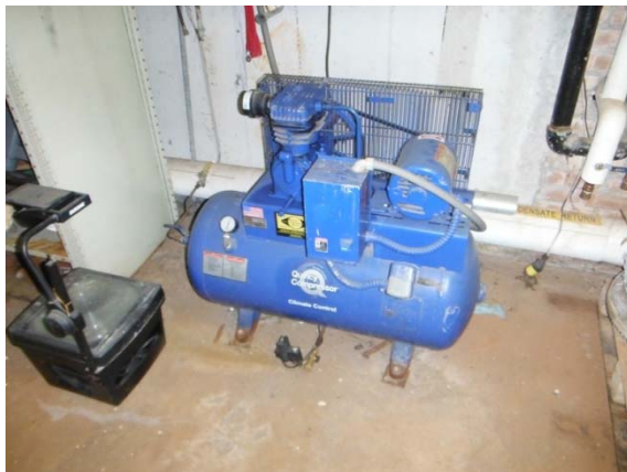
Photo #41: HVAC air compressor
