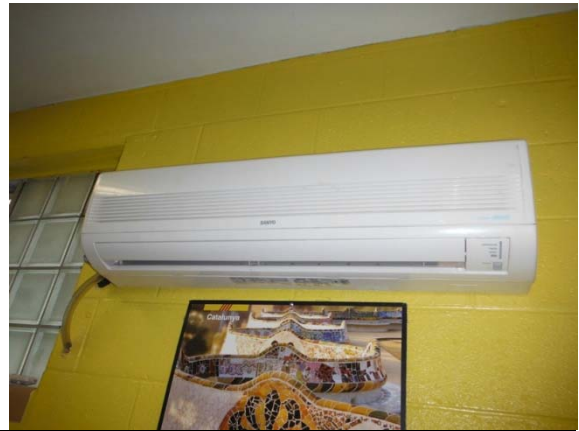
Photo #50: Ductless air handler in Parent liaison office
