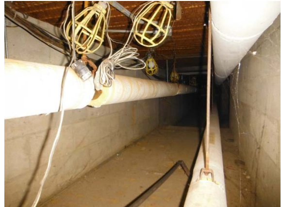
Photo #40: HVAC tunnel serving original building sections
