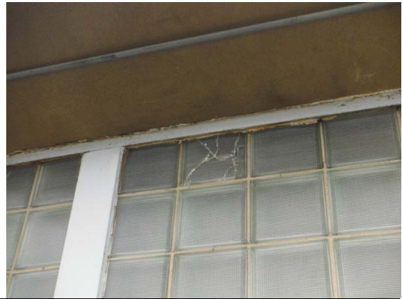
Photo #68: Cracked glass block at original section of building
