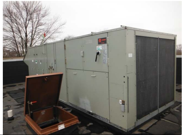
Photo #44: Gas-fired RTU for 2005 building addition
