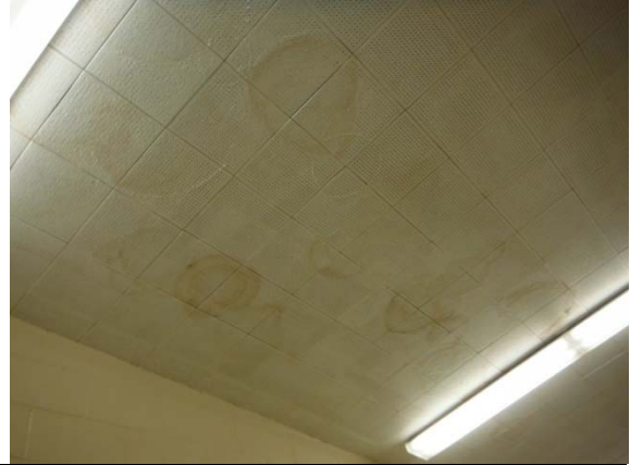
Photo #80: Water stained ceiling tiles at classroom 301
