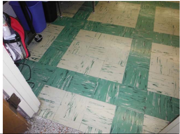
Photo #62: 9X9 suspect ACM vinyl tile in classroom of original building section
