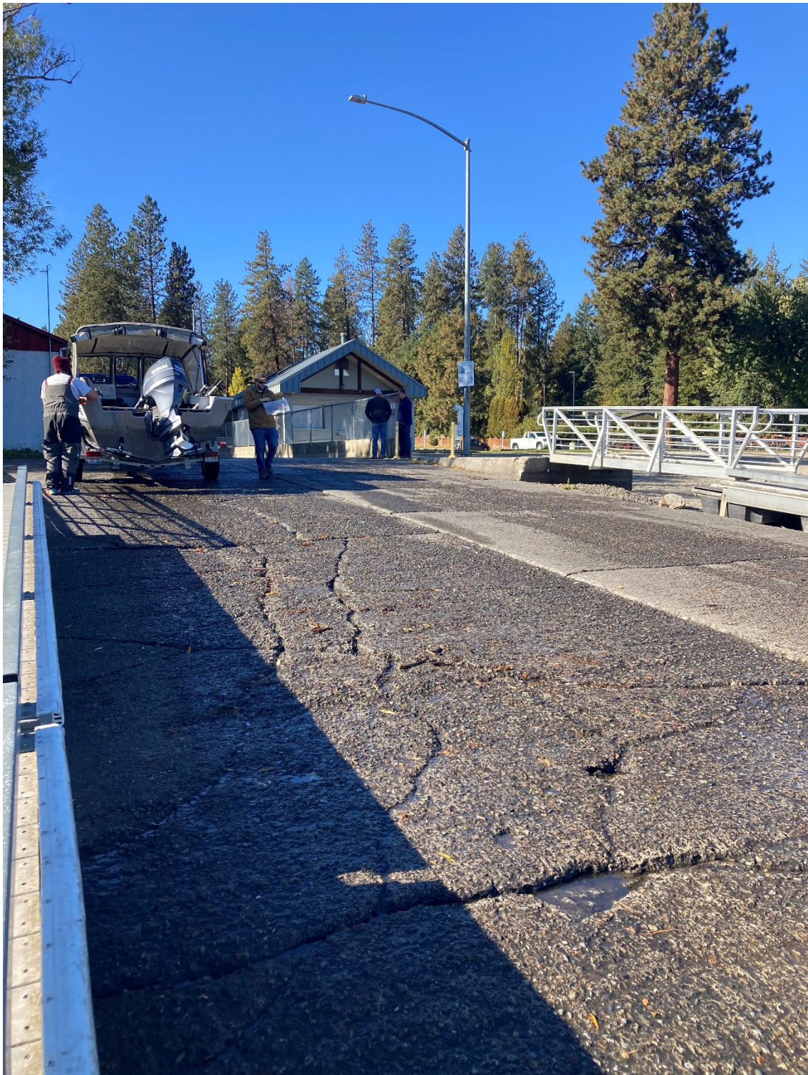
Honeysuckle Ramp Concrete
