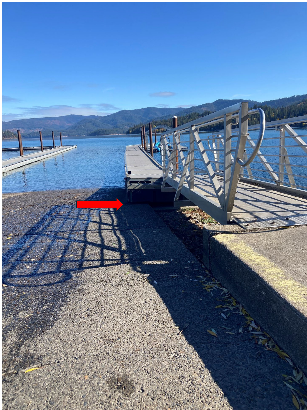
Honeysuckle South Dock Resting on Ramp
