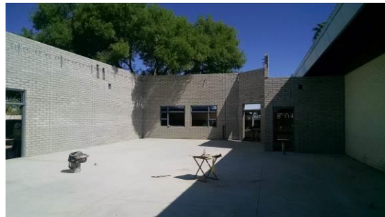
Block walls complete
