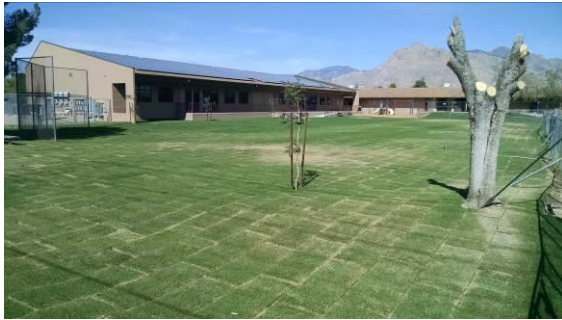
South side of New Building
