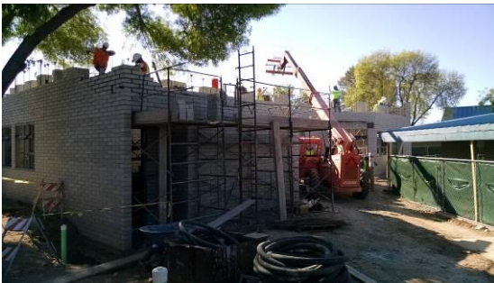
Block walls in progress
