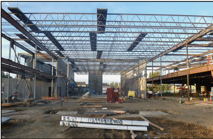
Trusses over gym
