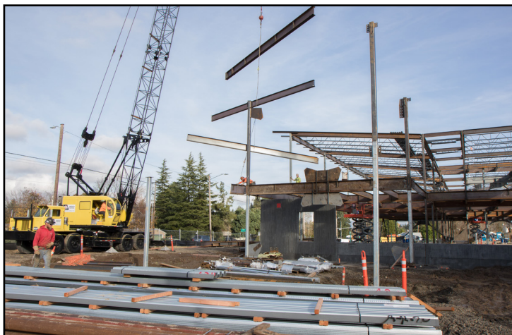
Steel beams in administration area
