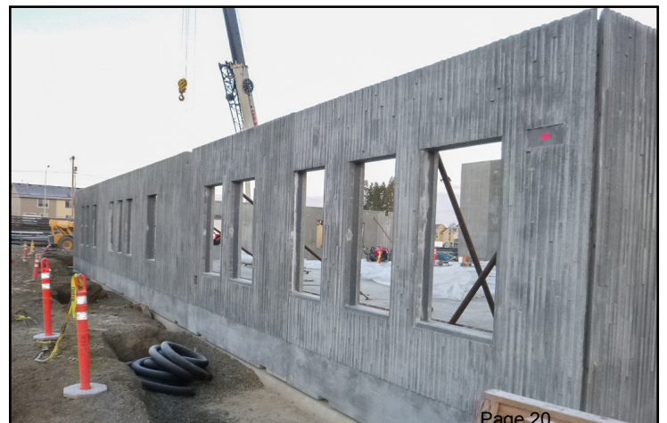
Precast panels in administration area
