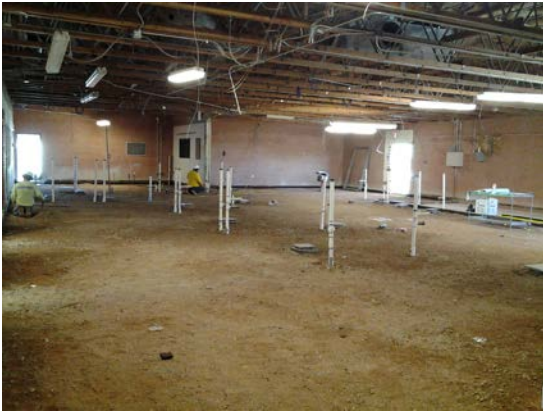
Kitchen Underground Prep for New Slab
