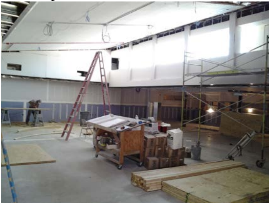
Library Drywall and Millwork Installation
