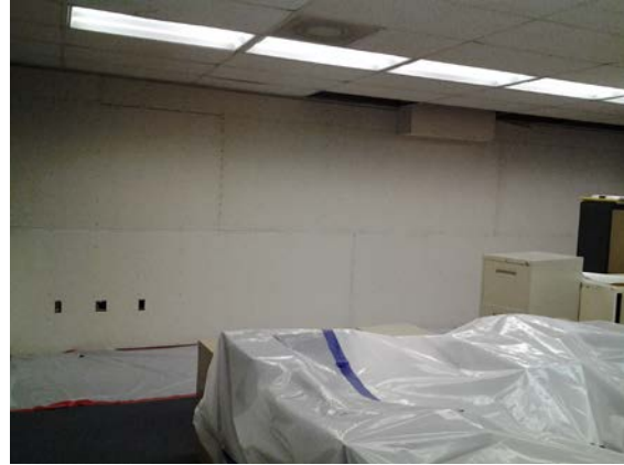
New Classroom Walls Framing, Infrastructure, and Drywall
