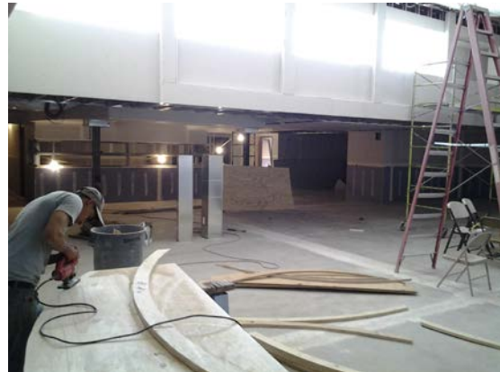
Library Drywall and Millwork Installation
