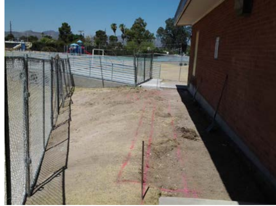
Layout for New ADA Ramp to Comp Lab
