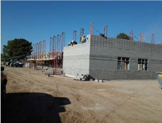
New Classroom Building Exterior Masonry Walls
