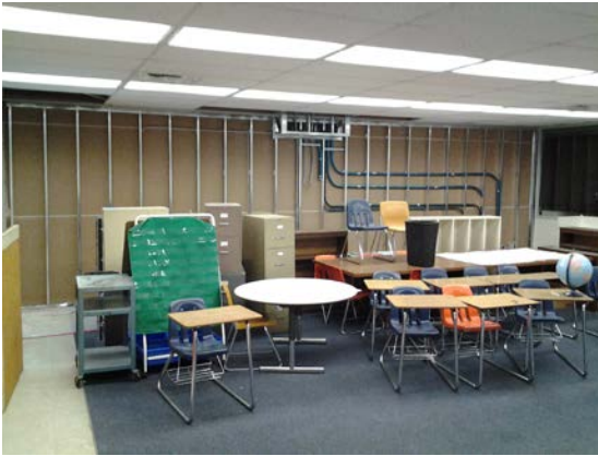
New Classroom Walls Framing, Infrastructure, and Drywall
