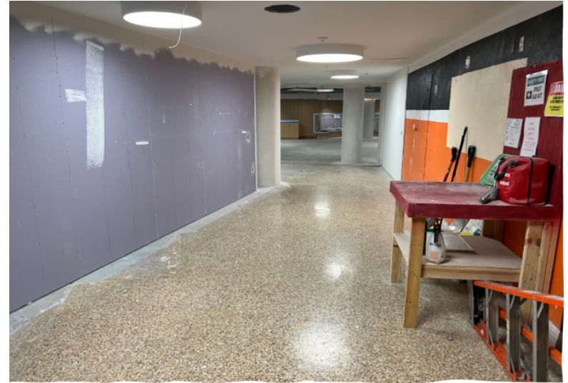
Current - SE entrance to Media Center
