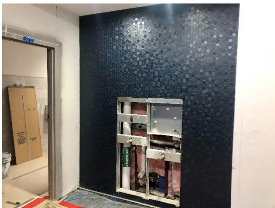
Tile on 2 nd Floor Rest Room in South Building
