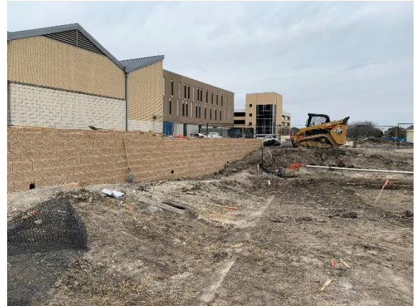
Retaining Wall, North of Alumni Hall
