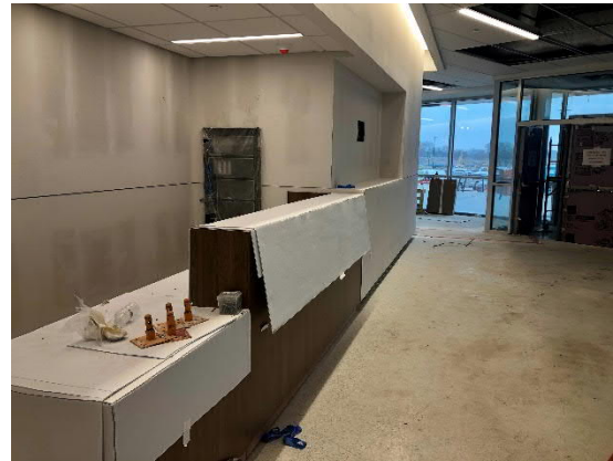
Information Desk at Main Entrance of North Building
