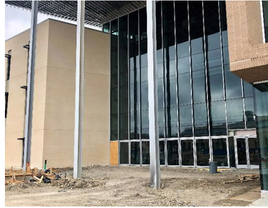
Main Entrance to Atrium
