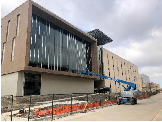
NE View of Building
