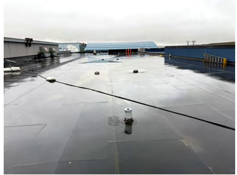
Completed EPDM roofing system with drainage swells and positive flow drainage that the school did not have before.
