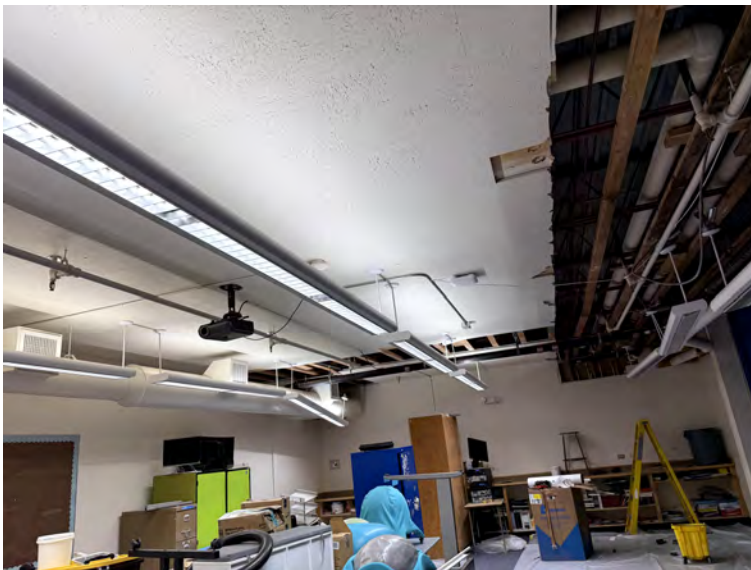
Interior ceiling tile and sheet rock demolition for roof drain pipe additions.
