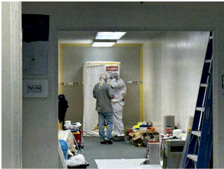
Asbestos remediation employee preparing to enter closed forced air enclosure.
