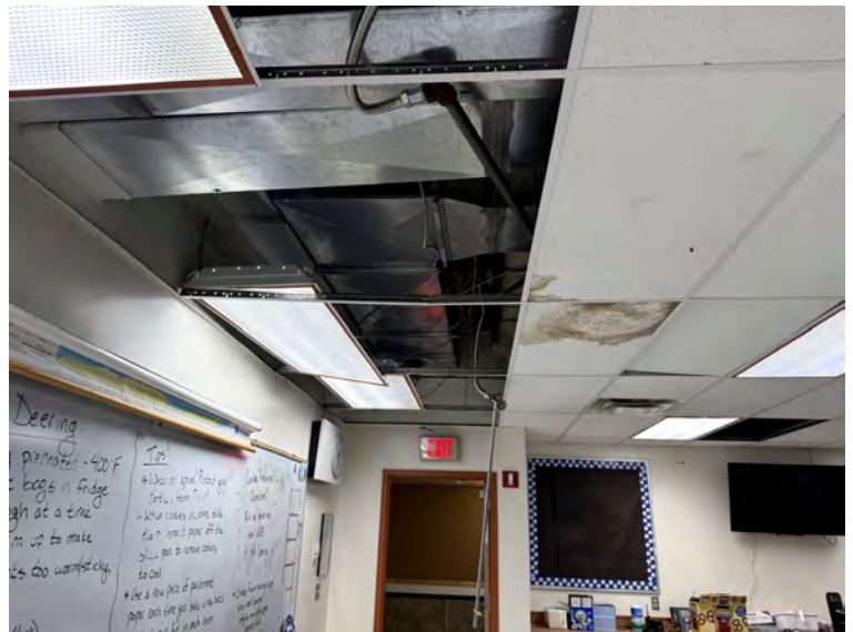
Ceiling tile removal for mechanical access for additional piping installation.
