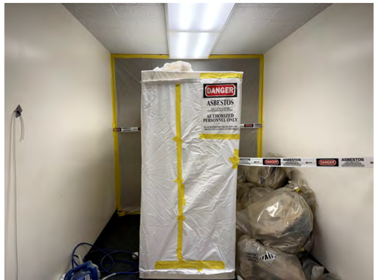
Asbestos remediation area enclosure with bagged asbestos.
