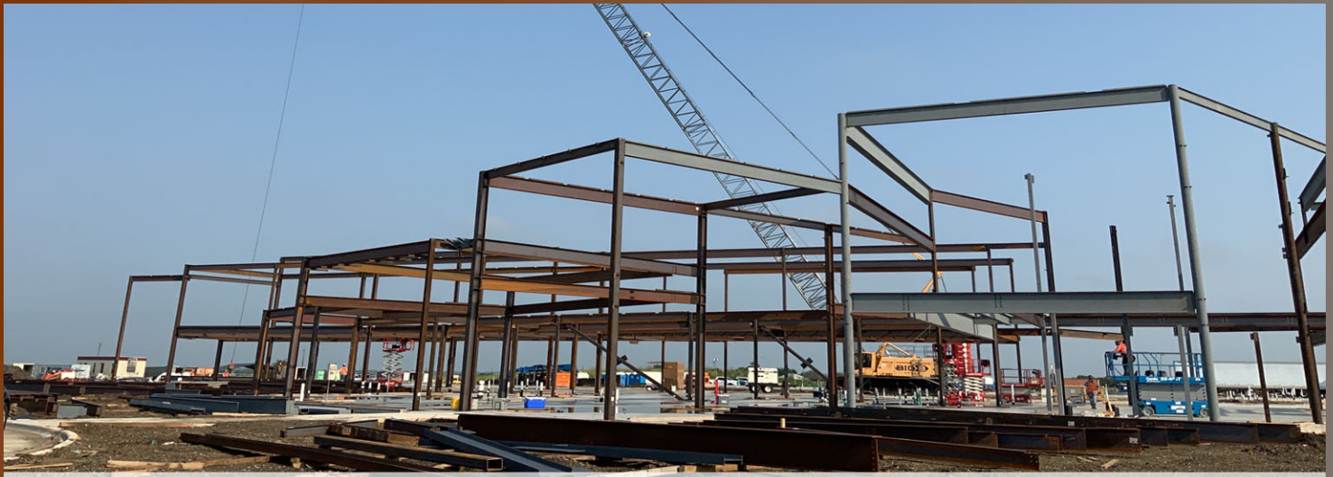
STRUCTURAL STEEL INSTALLATION
