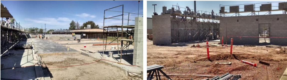
Slab on Grade and Exterior Concrete Masonry Block Installation
