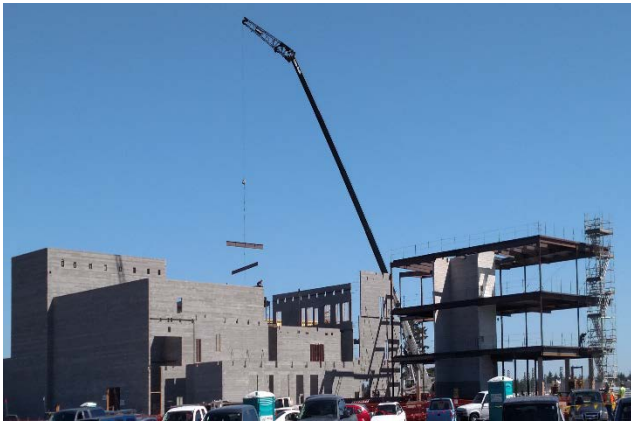
Steel going into Auditorium - looking southeast
