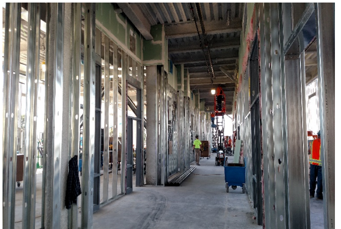
Classroom wing framing
