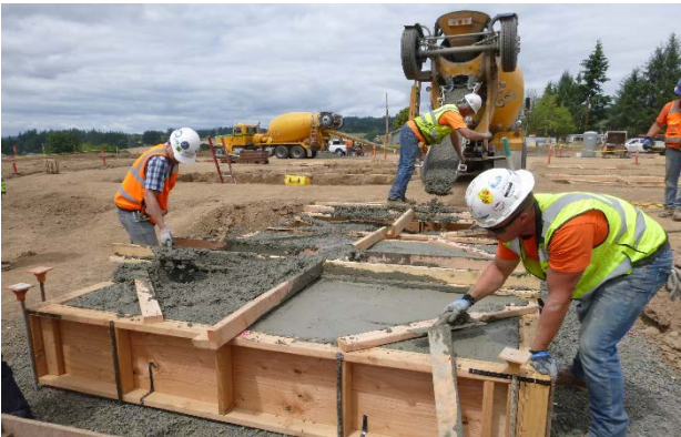
Concrete footings - looking northeast
