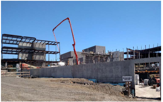
Administration/Auditorium - looking northeast
