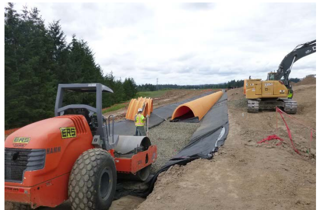
Storm water system - looking west
