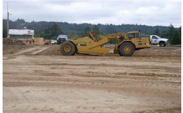
Parking lot scraping - looking northwest
