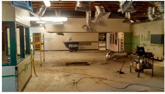
Library: The library has been evacuated and is undergoing interior demolition for installation of new shelving, a new circulation desk, and enclosure of the computer lab to
