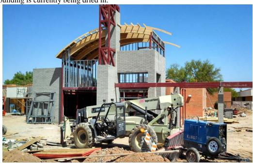
New Classroom Building: Drywall is complete. Ceiling tile and mechanical finishes are being installed. Exterior doors, windows, and paint are being applied.
