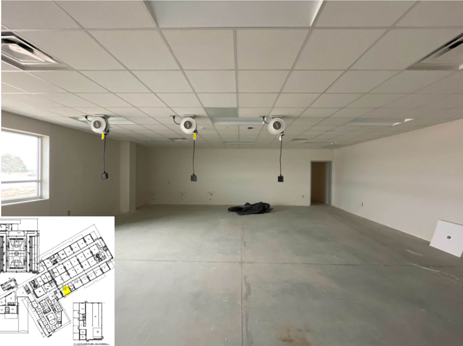
Classroom Wing Area A/A1
