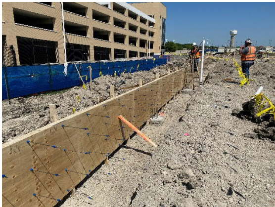
Exterior Grade Beam Formwork Install
