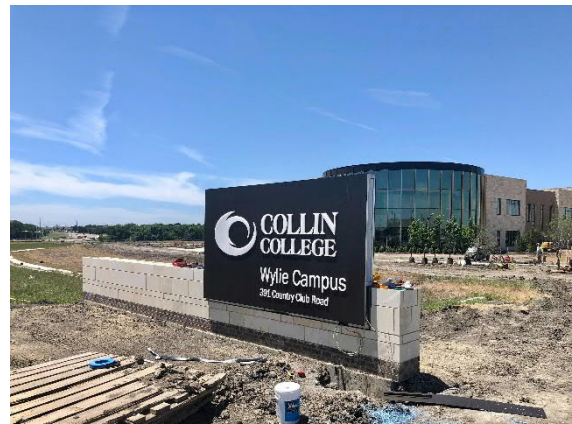
North Entrance Monument Signage Installed
