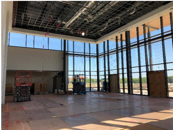
Conference Center Lobby/Pre-Function Area
