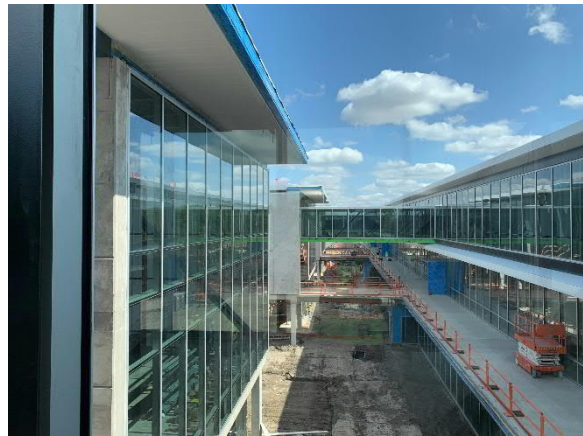
Northeast View of Trade Bar C Bridge
