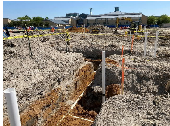
Underground Plumbing Install
