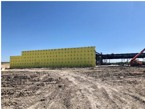
Sheathing of Office Lab Space
