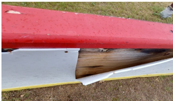
15: Damaged rink dasher boards
