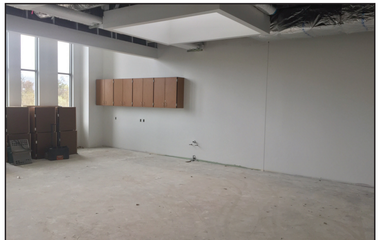
Classroom casework and painting
