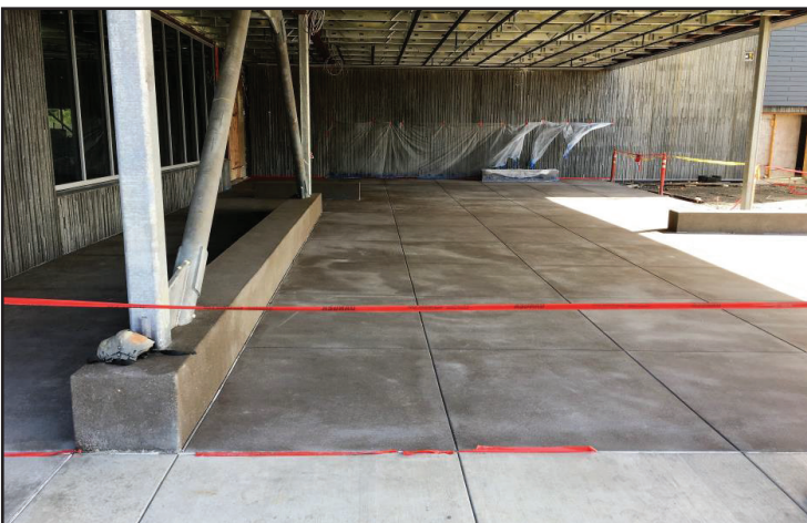
Colored concrete at West Entry
