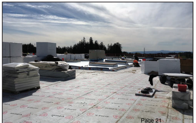
Roofing above Gym
