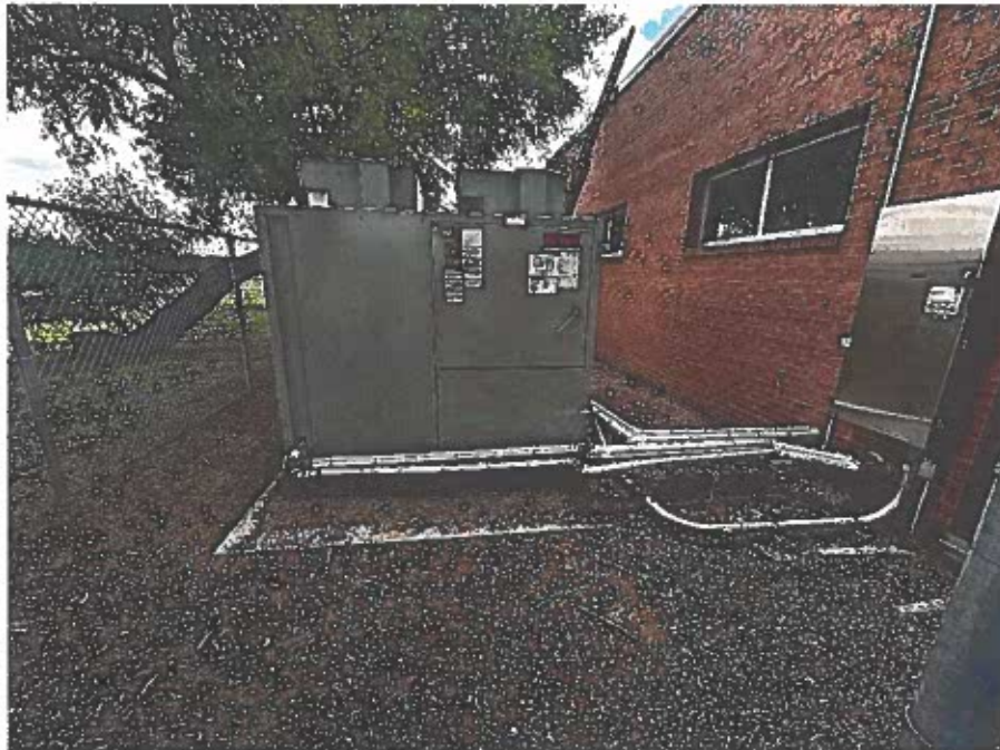
7. Adjust supports so that there are no sags or bending in the pipes. Pipes should look straight.
