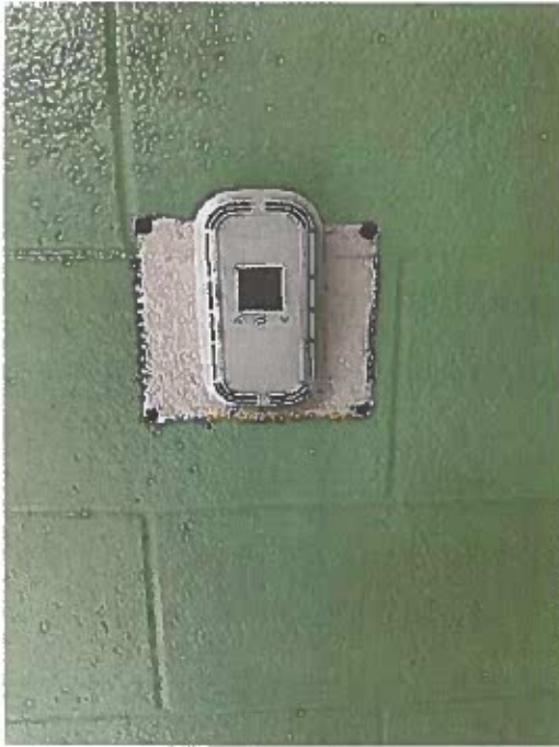
26. Cover holes and touch up with paint to match wall where existing thermostat was located.
