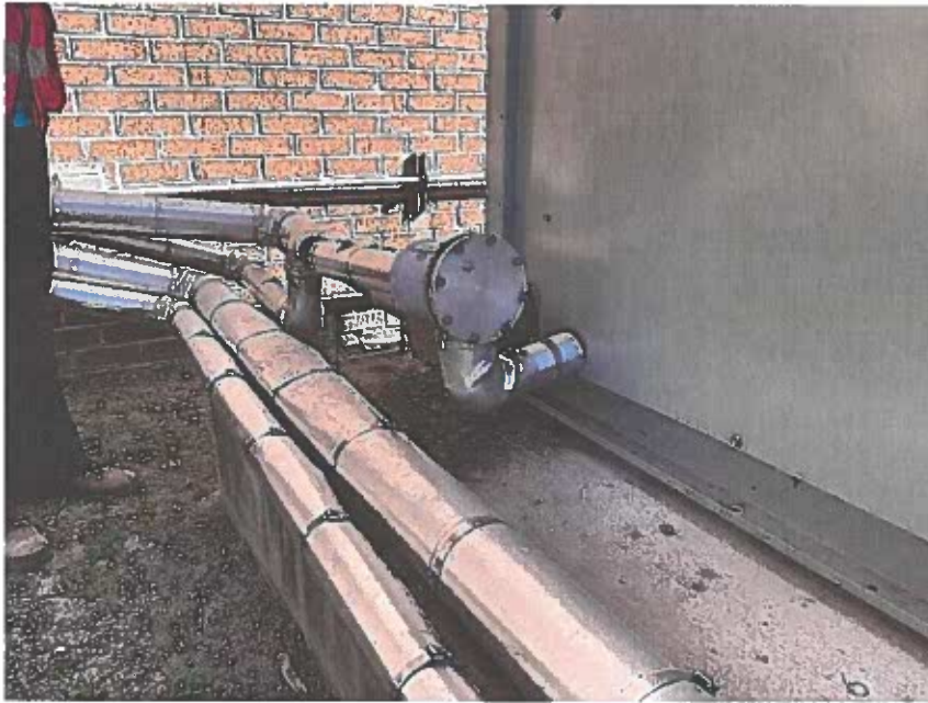
40. Replace damaged aluminum jacketing.
