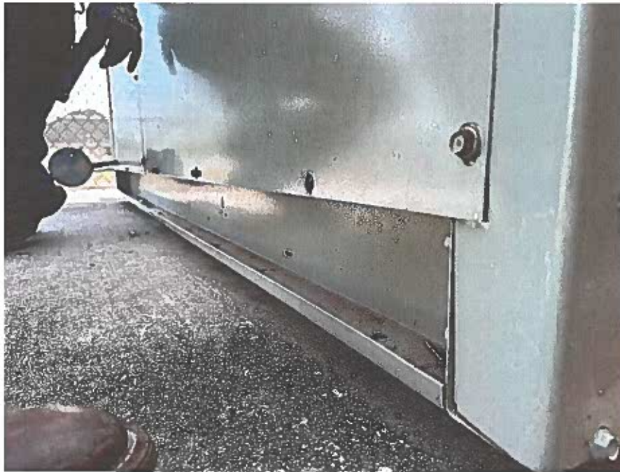
6. Install missing fasteners.
