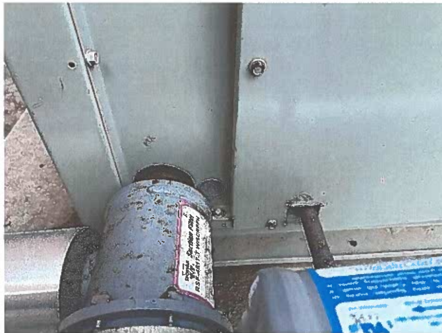
5. Seal piping penetration to condensing unit. Typical.
