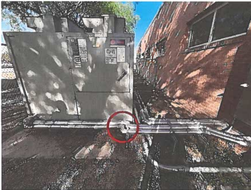
41. Fasten loose piping clamp supports.
