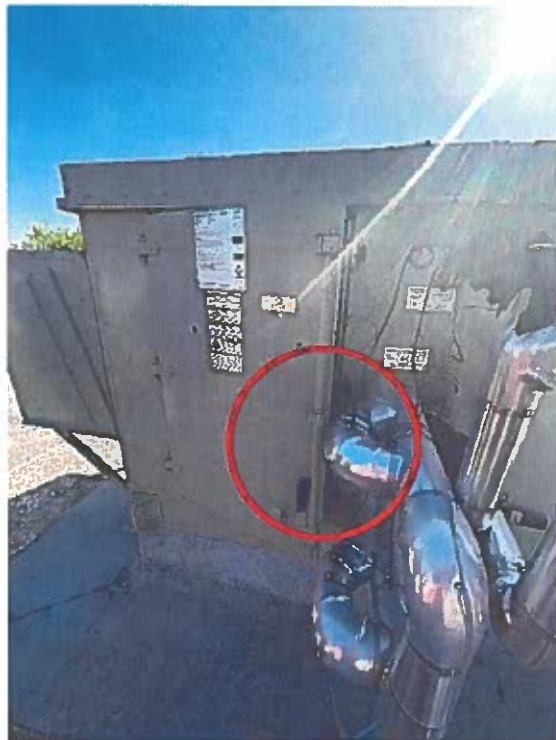
39. Adjust piping position to avoid conflict to open filter access.
