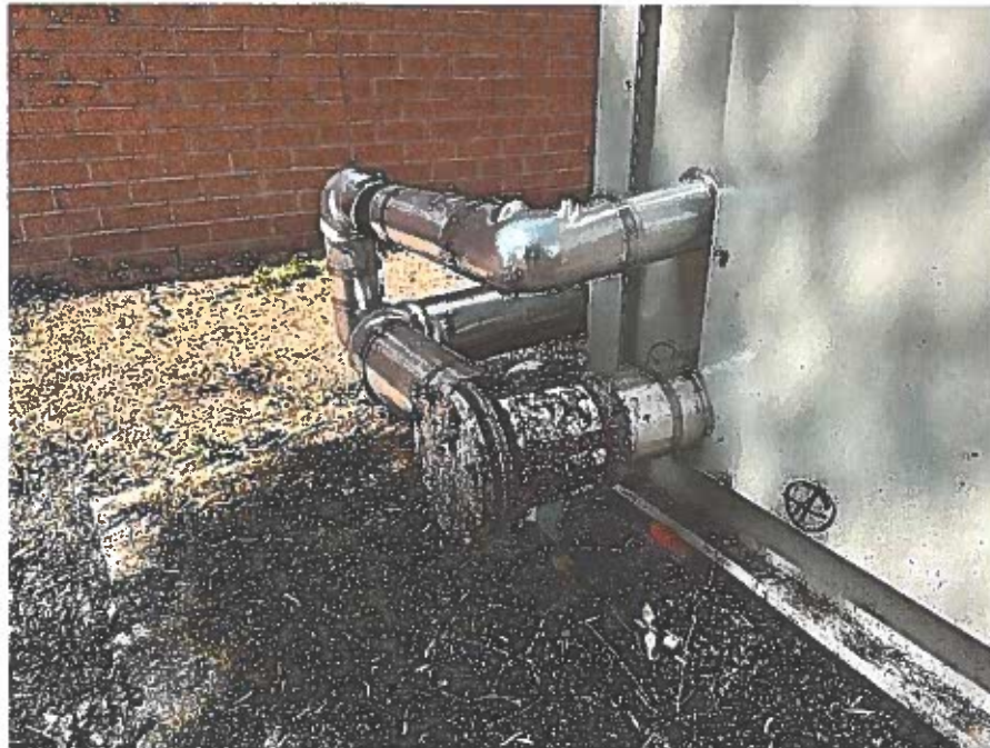
9.— Clean up debris from piping and suction filter.
