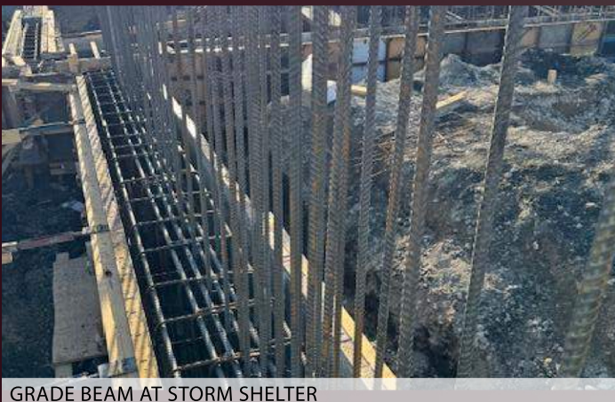
GRADE BEAM AT STORM SHELTER
