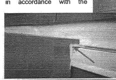
1.04 On the south side of the HVAC unit, the base flashing membrane has become disbonded and is open to moisture intrusion. This location was previoulsy marke for repair by the manufacturer's technical representative.
