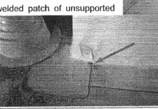
1.08 On Roof Area C, at the location of the elevated Condenser unit, one outside corner flashing was installed with a hole in the membrane. This is often the result of an over stretched membrane and could result in moisture intrusion into the roof system and ultimately the structure as a leak.
