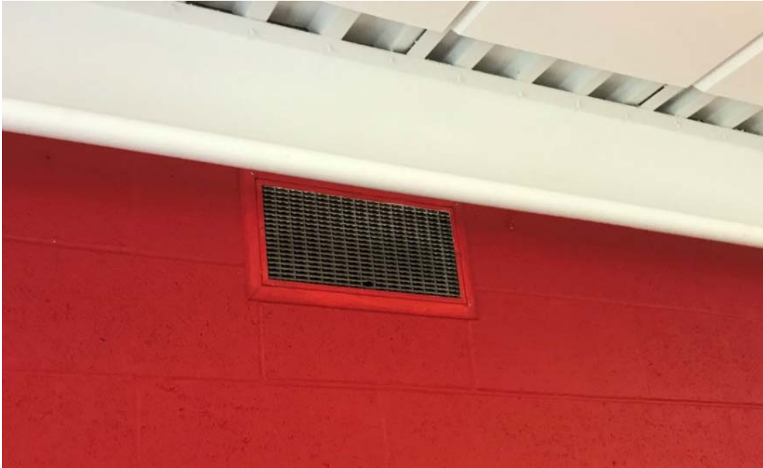
Figure 5- Typical Exhaust grill in classrooms with UV's
