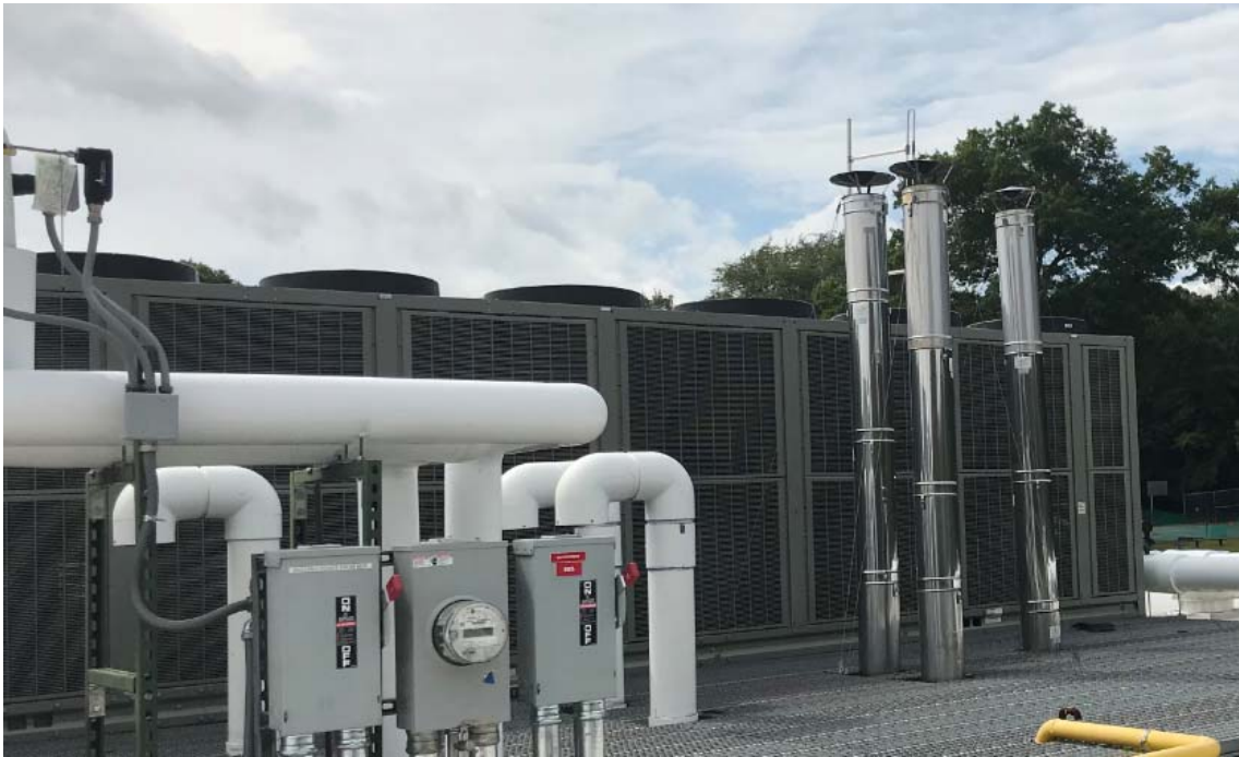
Figure 10-Roof mounted Chiller
