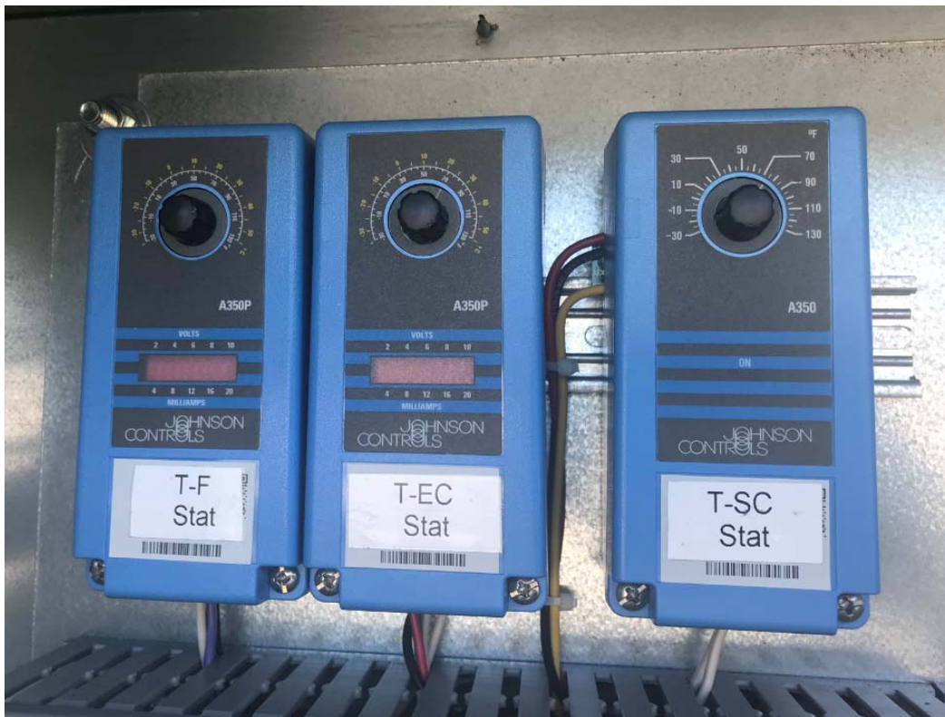
Figure 8- ERU local controls
