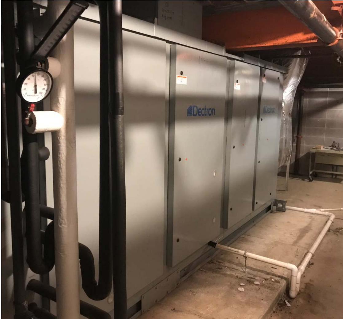
Figure 11-Dectron Unit serving pool
