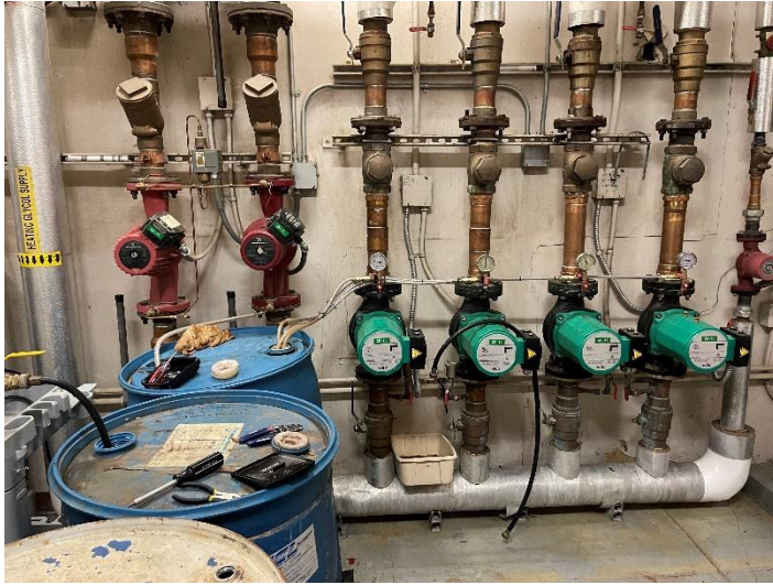
Photo M3 – Primary Heating Pumps
