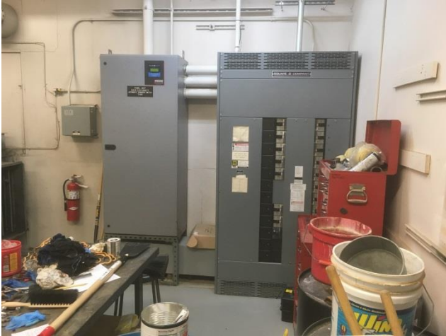
Photo E3 – Main Distribution Panel '2NMDP'
