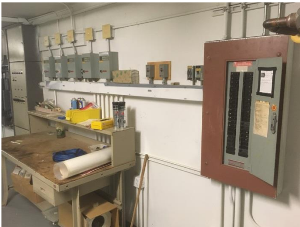
Photo E7– Older Panel and Motor Starters
