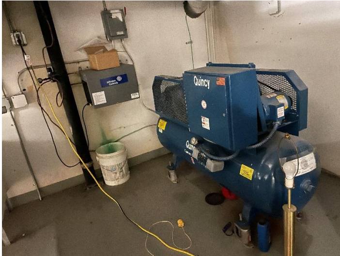
Photo M9 – Pneumatic Air Compressor
