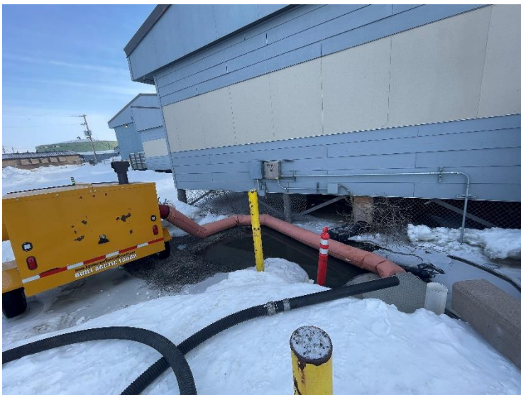
Photo M3 – Service Barrel Heating
