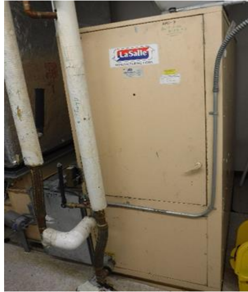
Photo M8 – Poor Condition AHU
