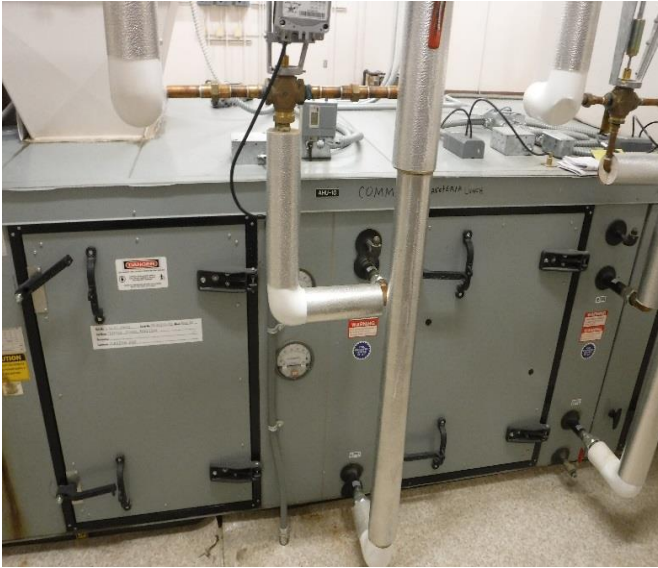
Photo M7 – Good Condition Air Handler
