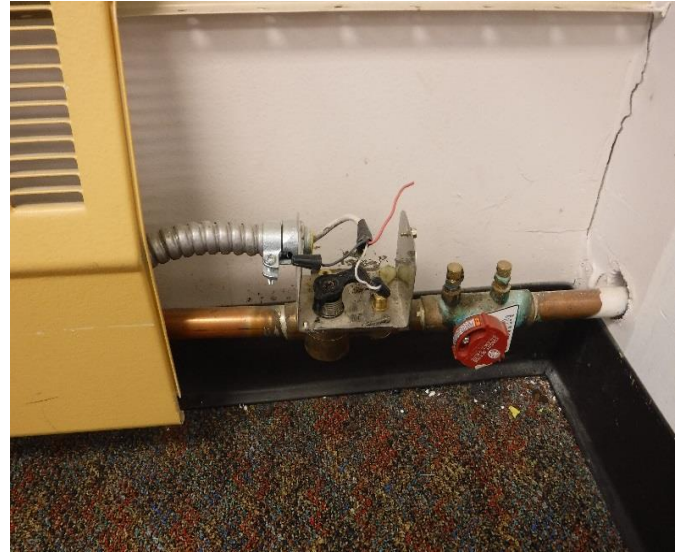
Photo M10 - Failed Finned Tube Valve
