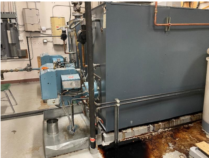
Photo M5 – Leaking Boilers
