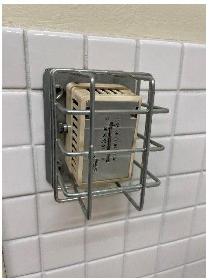
Photo M11 – Pneumatic Thermostat
