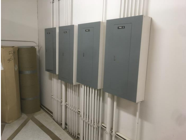
Photo E5 – Typical Panelboards (1997 remodel)
