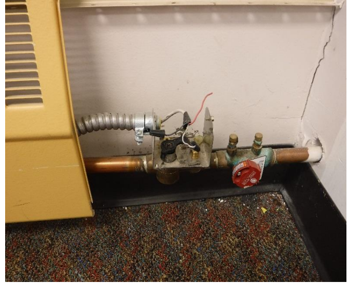
Photo M4 - Failed Finned Tube Valve
