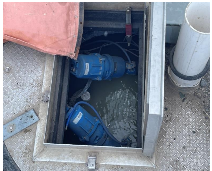
Photo M4 – Service Barrel Flooding
