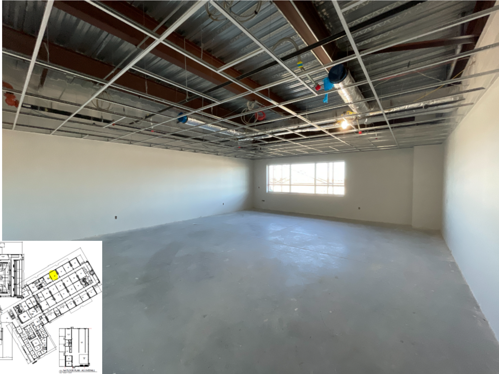
Classroom Wing Area A/A1
