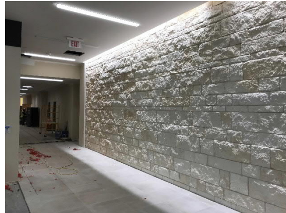
Interior Stone Wall in Lobby
