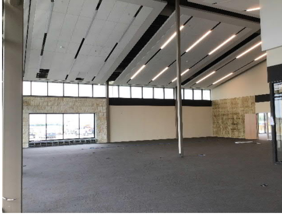
Carpet Installed at Library
