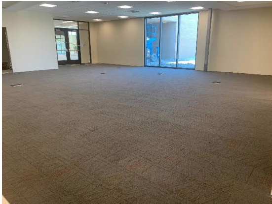
Carpet Installed at One-Stop Shop
