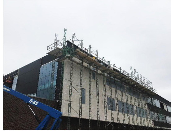
Block Work at East Elevation
