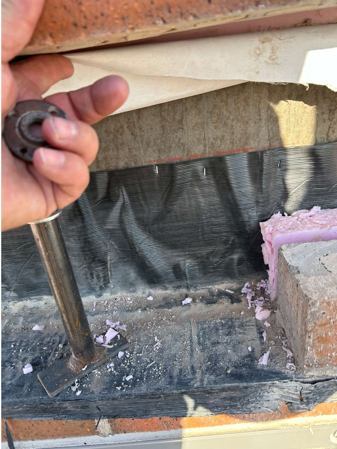
Original through wall flashing detail
