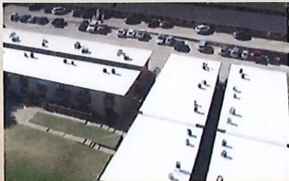
Silicone Roof Restoration -
