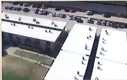
Silicone Roof Restoration -
