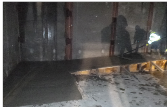
Freshly placed concrete
