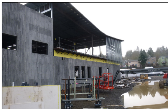
West facade of building
