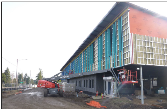
North facade of building
