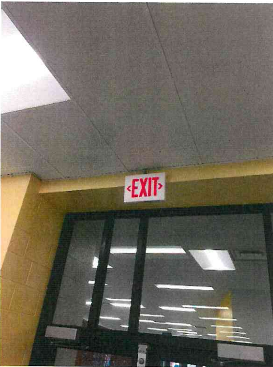
Exit sign to be installed to ceiling grid in cafeteria.
