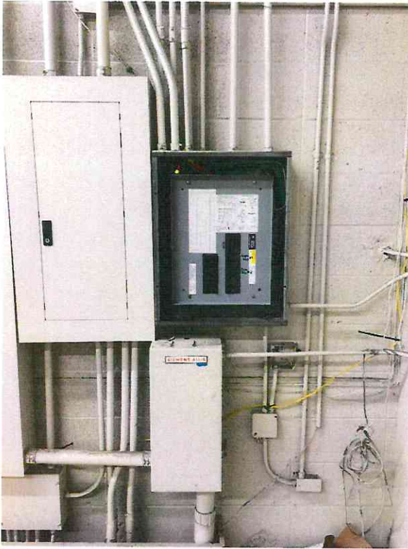
Install panel cover
