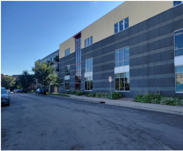
Existing School Exterior along Mercer Way
