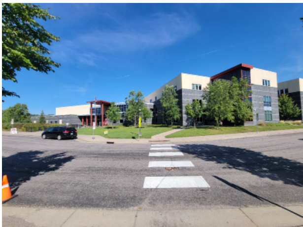
Looking towards Main Entrance from Public Parking along Victoria Way
