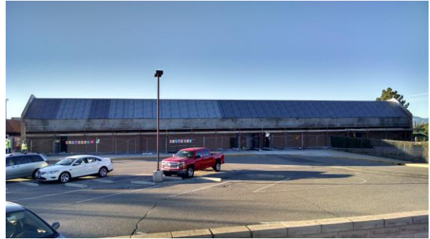
North Face of New Building
