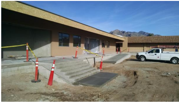
South Face of New Building
