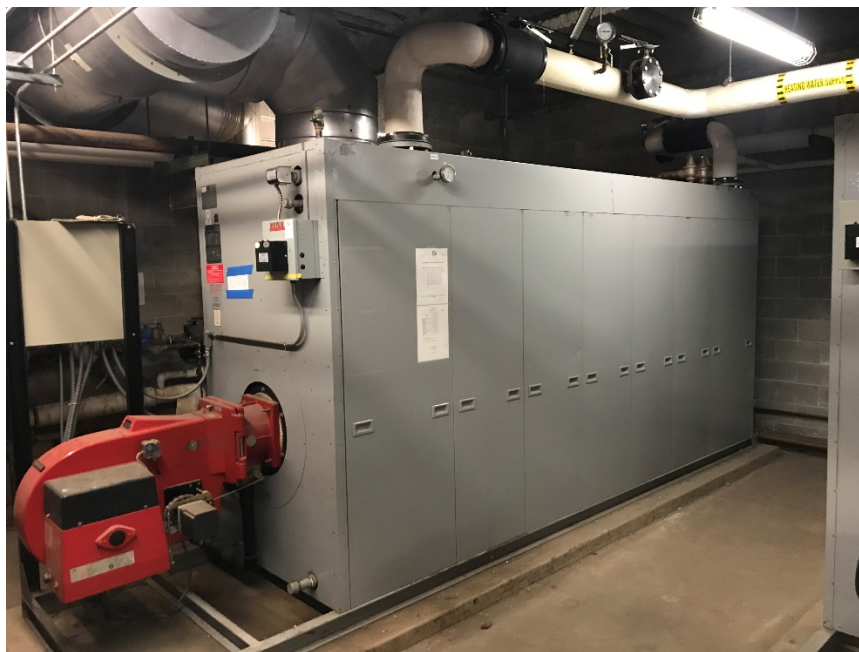
Figure 28: Bryan Boilers – (Space Heating Hot Water)
