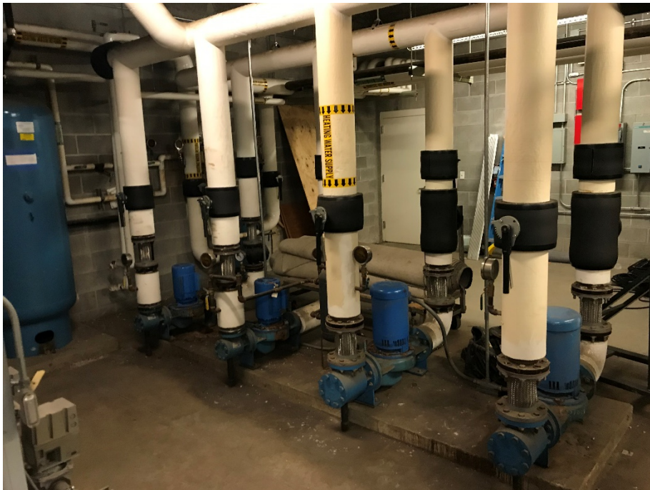
Figure 30: Space Heating Water Pumps
