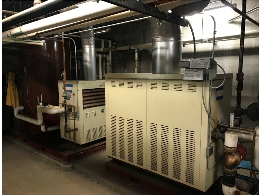
Figure 29: Tjernlund Boilers – (Domestic Hot Water)
