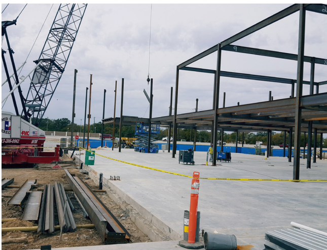
Steel Erection
