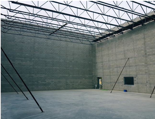
Band Hall CMU and Joist
