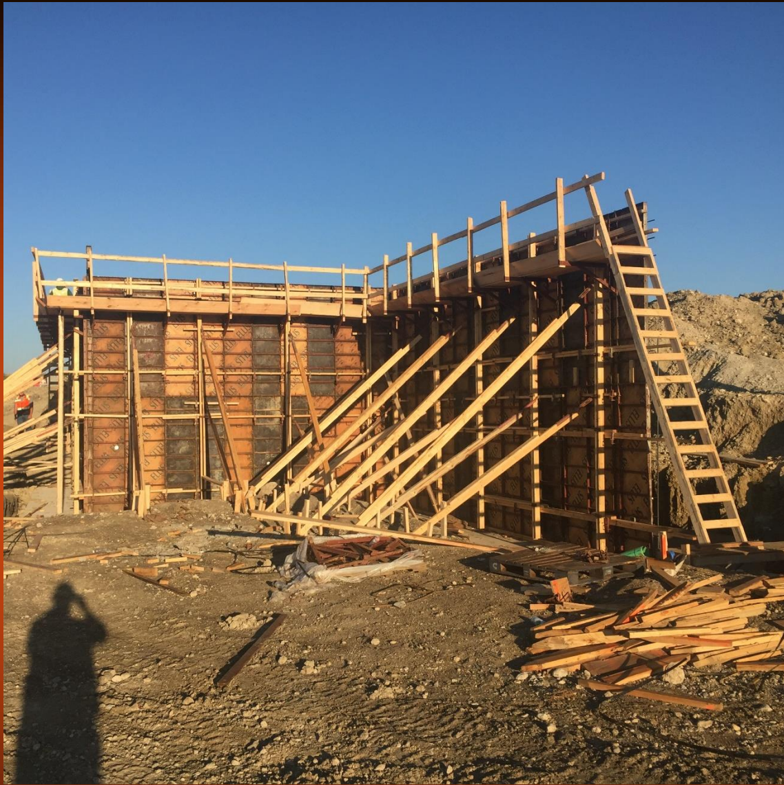
Elementary 5 Forms at South Retaining Wall
