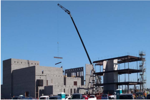
Steel going into Auditorium - looking southeast
