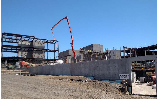
Administration/Auditorium - looking northeast
