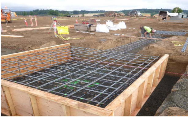
Footings - looking west
