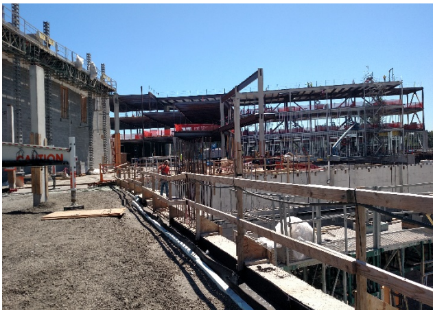
Commons/Classroom wing - looking east
