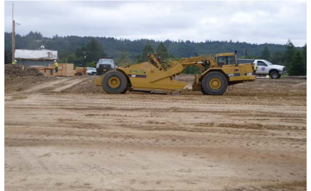
Parking lot scraping - looking northwest
