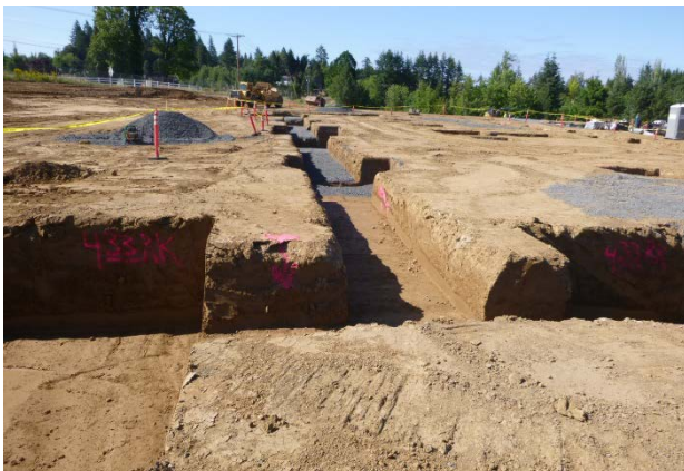
Footing excavation - looking northwest
