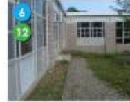
Rainwater Collection / Sustainability Garden Drainage Area 3 Priority: N/A Cost: N/A
