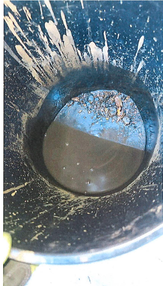
Adult Education fire sprinkler dry system ^
