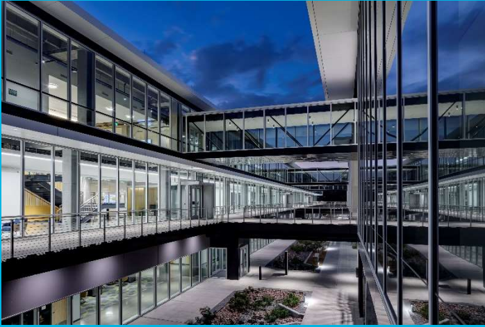
Bridges Connecting Academic Building Trade Buildings
