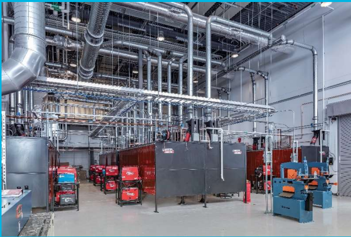
Welding Lab in Trade Bar B
