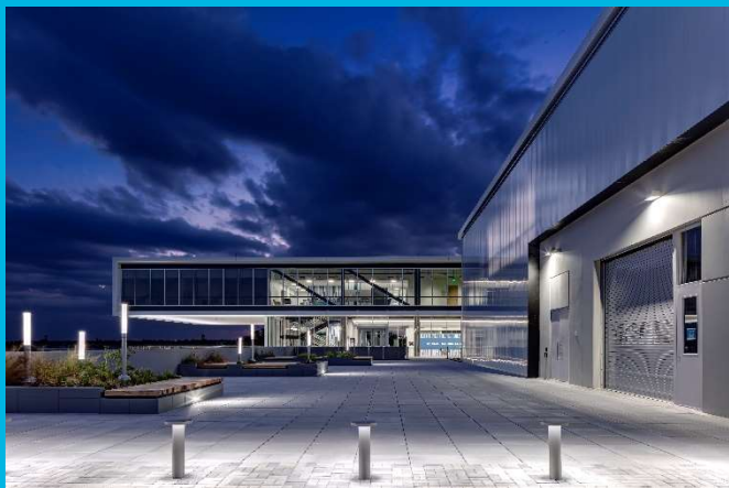
Campus Main Entry
