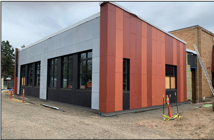
Northeast addition exterior siding
