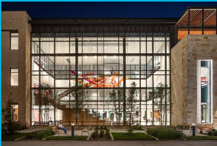
Curtain Wall at Student Center
