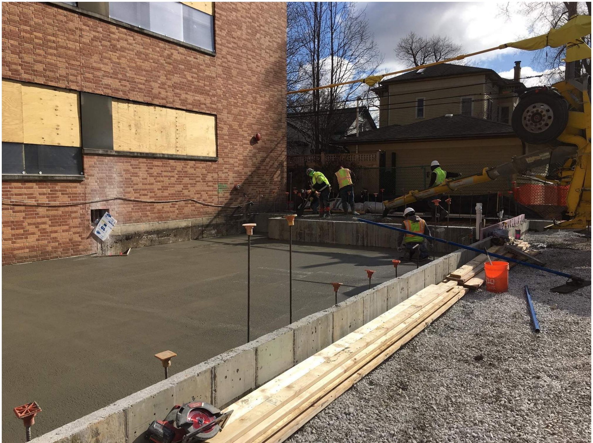
04/17/2018 - AREA B SLAB ON GRADE BEING POURED
