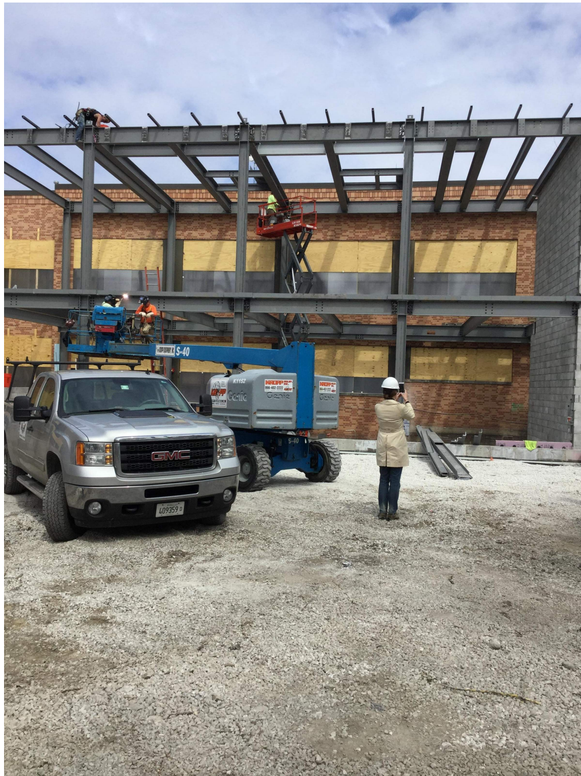
04/24/2018 - STRUCTURAL STEEL IN PLACE, STEEL DETAILING TAKING PLACE
