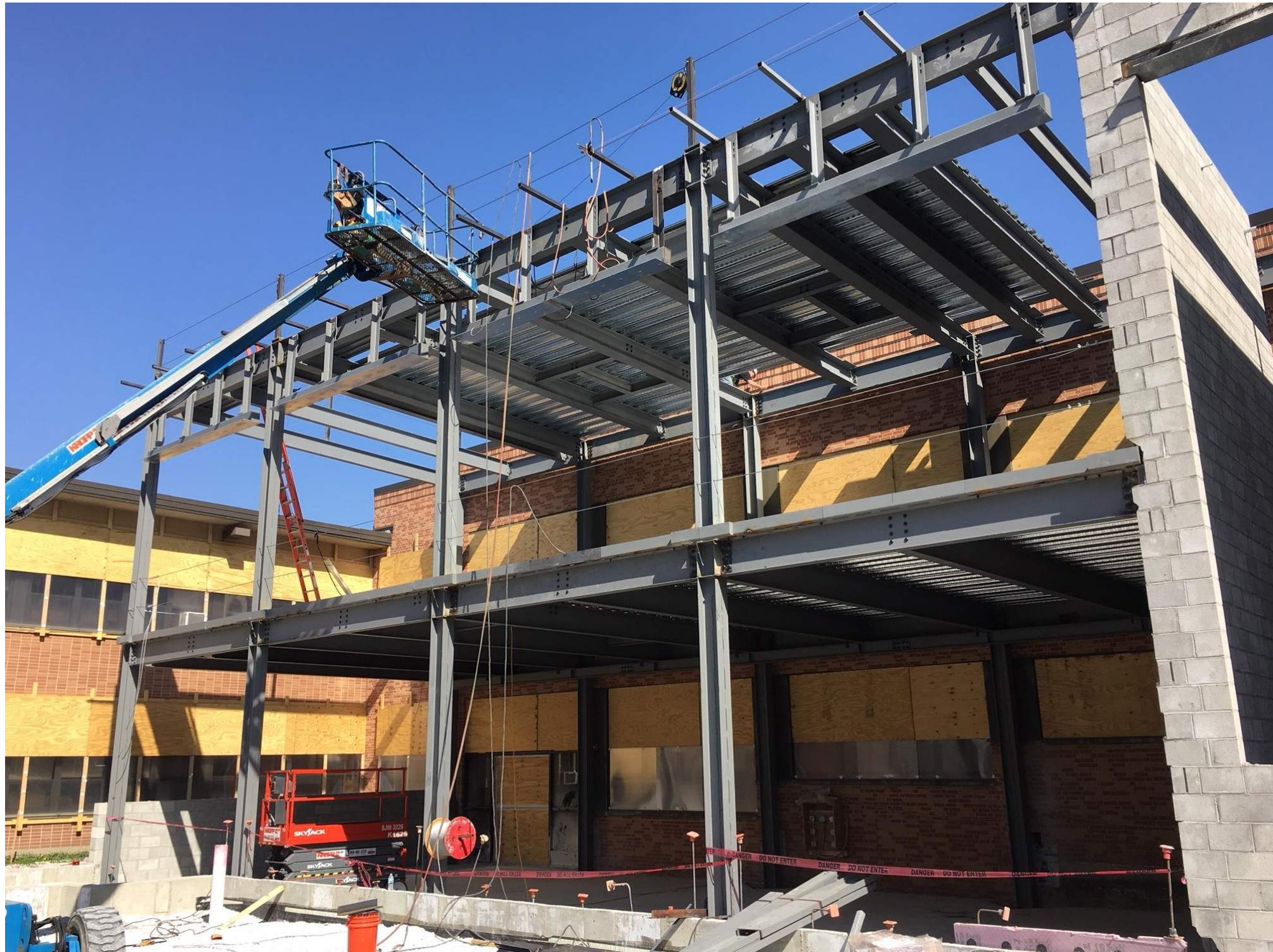
05/01/2018 - STEEL DECKING INSTALLATION
