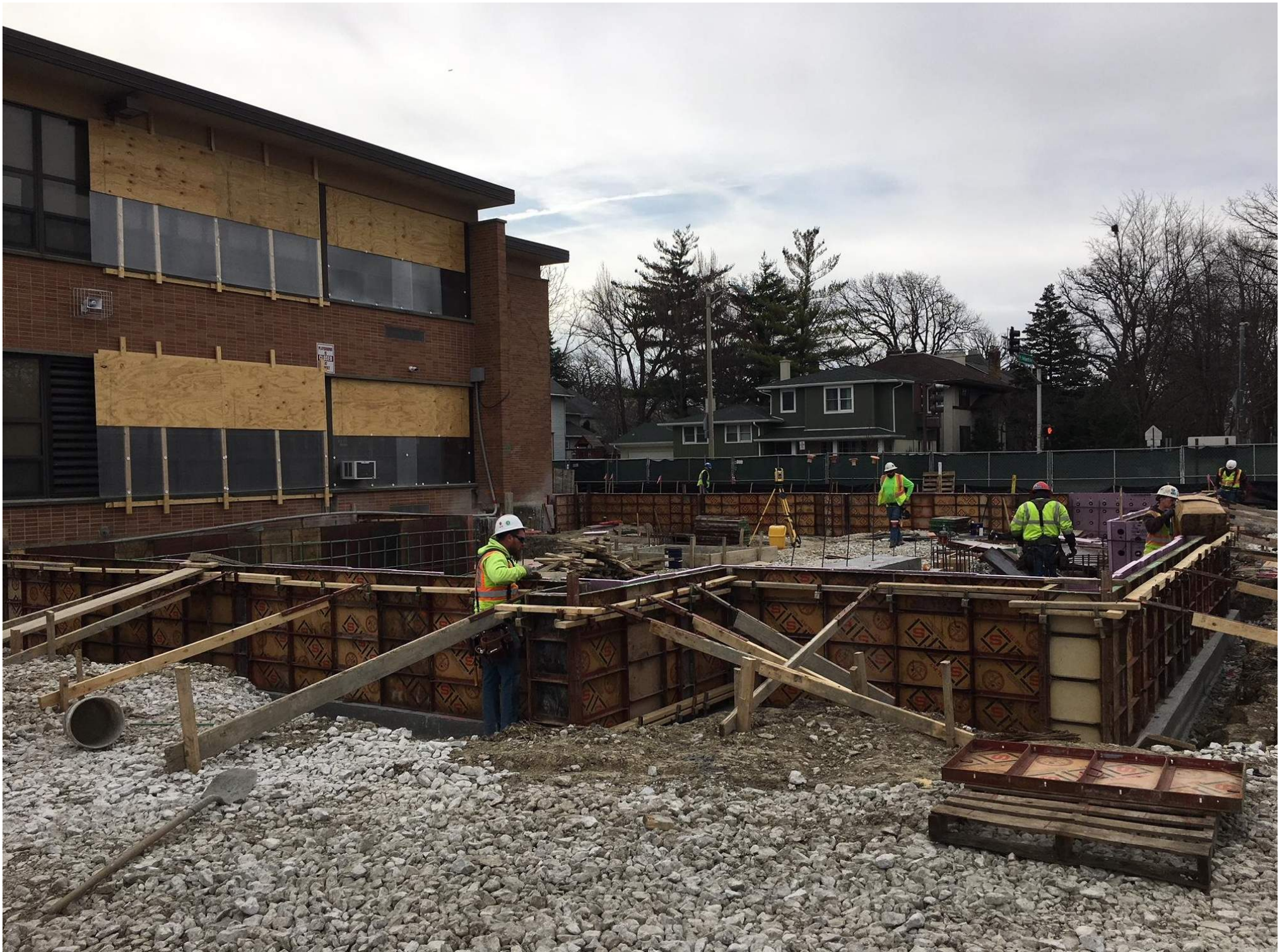
04/23/2018 - AREA A FOUNDATIONS BEING FORMED
