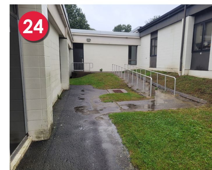
Revegetate Slopes Rain Garden Drainage Area 5
