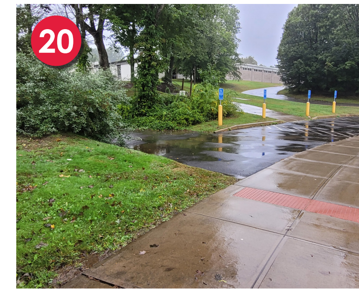
Revegetate Slope Drainage Area 4
