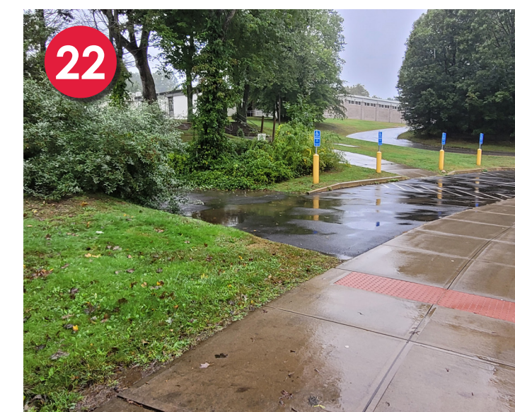
Pervious Pavement Drainage Area 4
