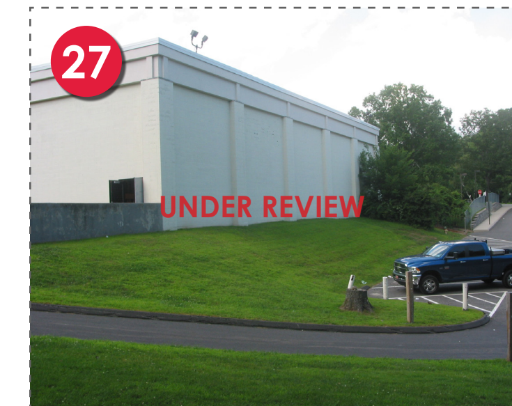
Revegetate Slope Drainage Area 6
