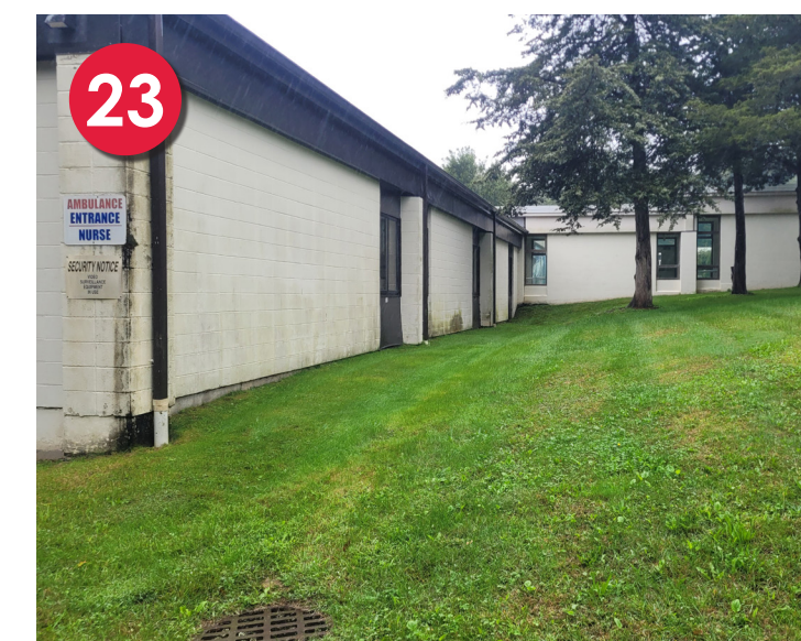
Rain Garden Drainage Area 5
