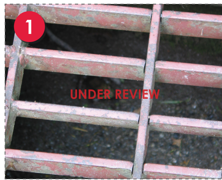
Catch Basin Cleaning Energy Dissipater Outfalls All Drainage Areas
