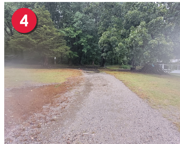
Biofiltration Swale Drainage Area 1
