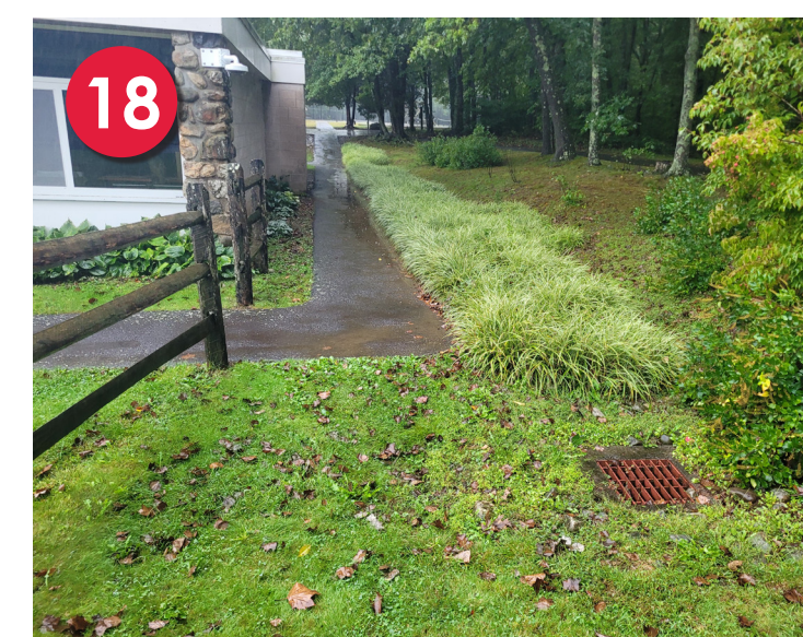
Rain Garden Drainage Area 1 & 2
