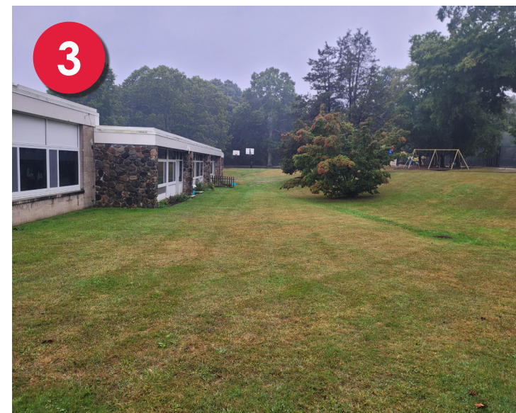
Rain Garden / Retention Basin Drainage Area 1
