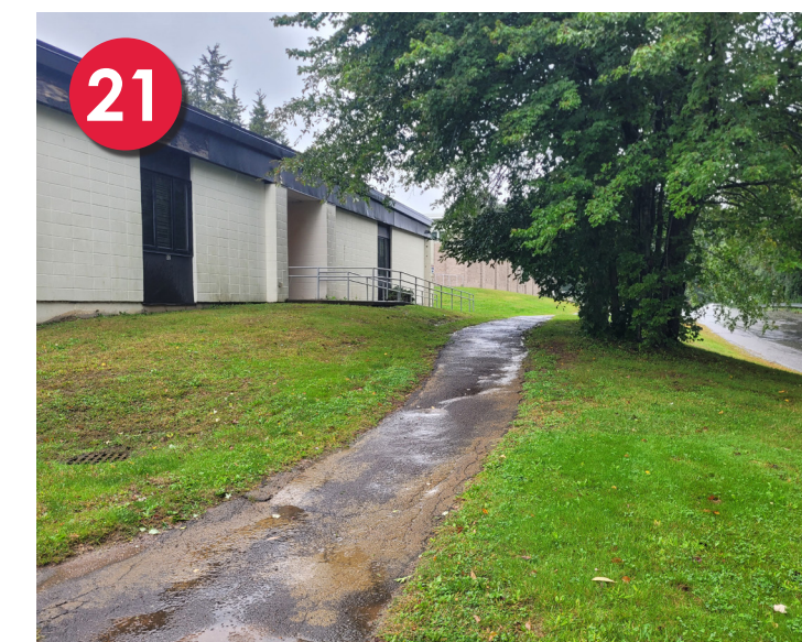
Biofiltration Swales Drainage Area 4
