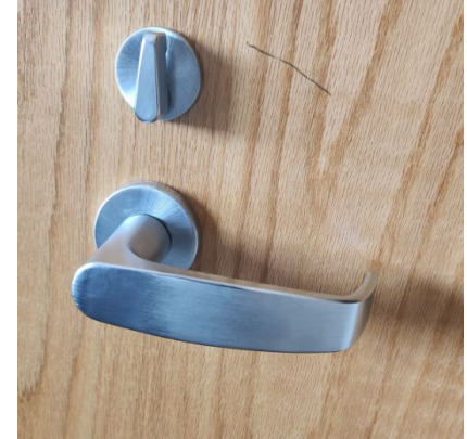
Mortise Thumb Drive Lock (Most Common on Office Room Doors)
