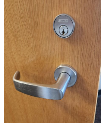
Mortise Thumb Drive Lock (Most Common on Office Room Doors)
