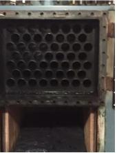
Soot shown in picture comes from build up from incomplete combustion. Causing carbon monoxide within boiler room on March 4,2018. After Maintenance Mike Bowens turned off both furnaces. Firefighters and gas company worked to ensure carbon monoxide was clear from school 1st floor to ensure safety for school to start on March 6,2018. (Note 1800 was the level of carbon produced well beyond legal for facility) Bryant Boilers deaned on March 5,2018 and March 7, 2018.
