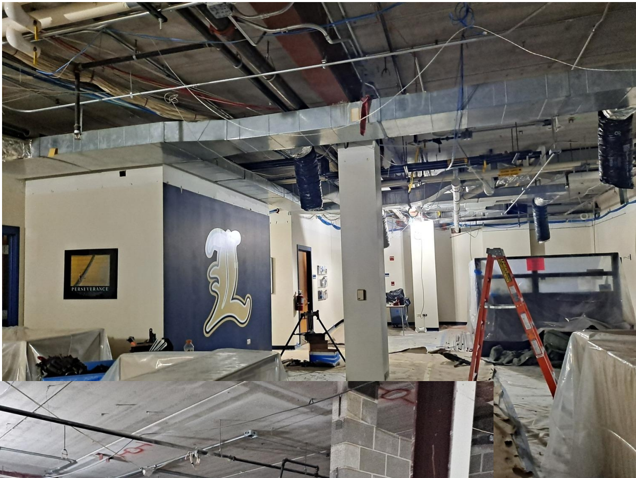
FIRST FLOOR OFFICE CEILINGS REMOVED FOR SCIENCE PIPING ABOVE
