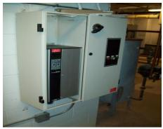
Variable Frequency Drive (VFD) VFDs have started failing this year. All units need replacing.
