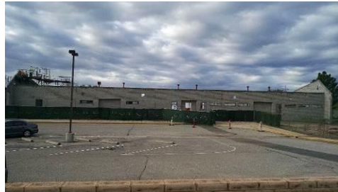
The North Side of New Building
