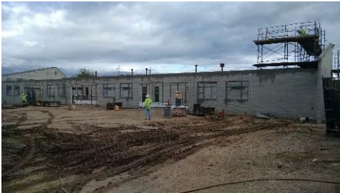
The South Side of New Building
